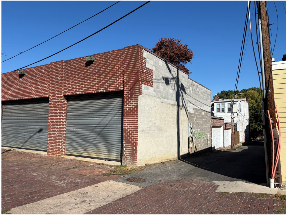
EXISTING GARAGE AT 1223 F STREET NE
