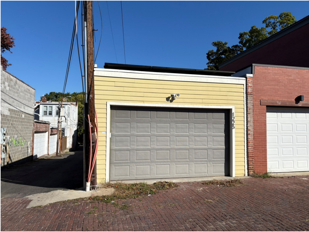
EXISTING GARAGE (SOUTH VIEW)
