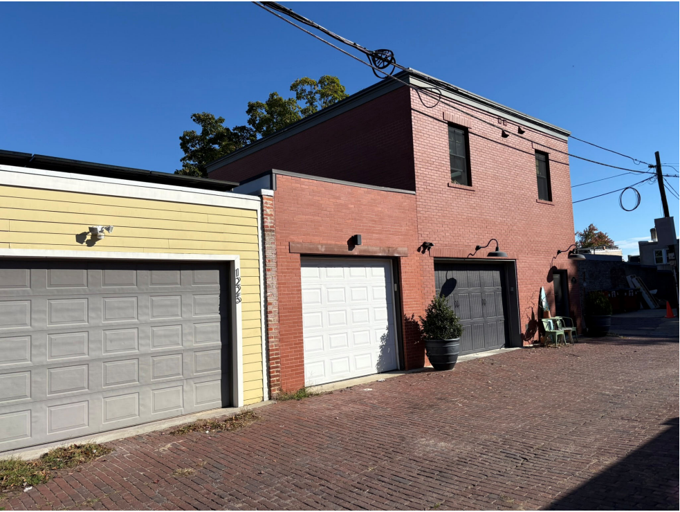
EXISTING GARAGES TO EAST
