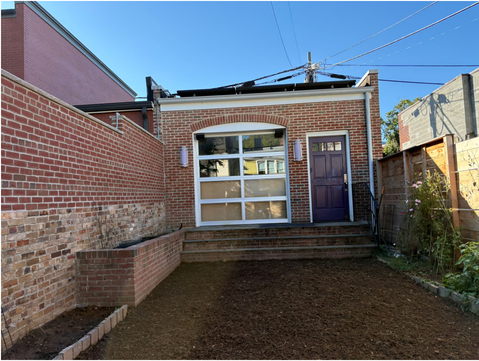
EXISTING GARAGE (NORTH VIEW)
