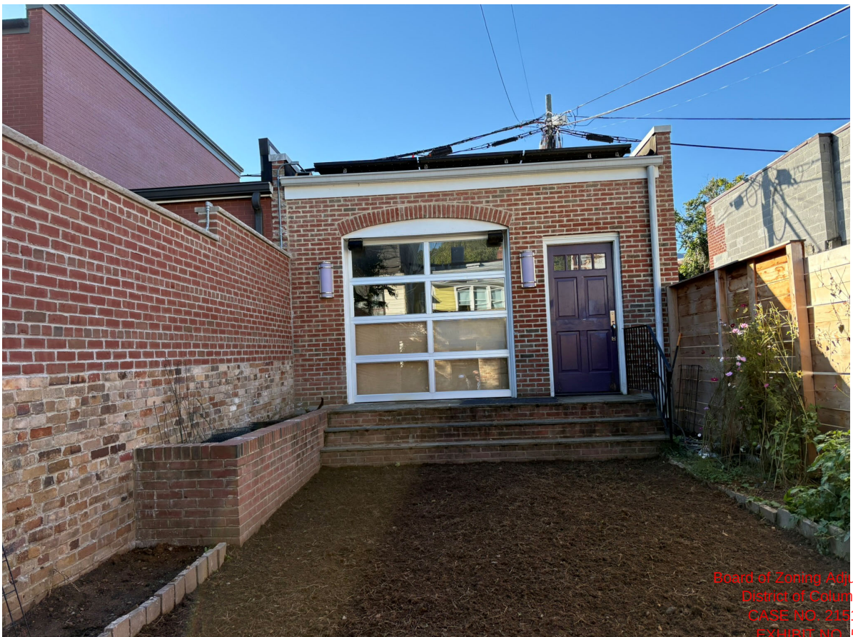
EXISTING GARAGE AT 1225 F STREET NE
