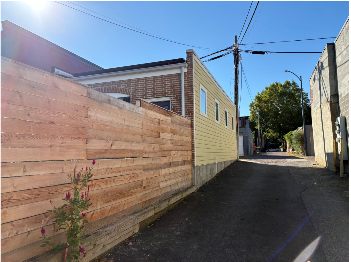
EXISTING GARAGE AT 1225 F STREET NE
