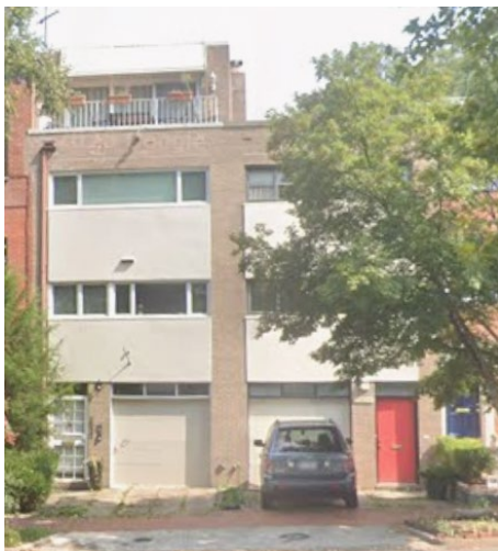
Asymmetrical massing on the Property, which is missing the fourth floor and no longer provides bilateral symmetry with the adjacent home.
