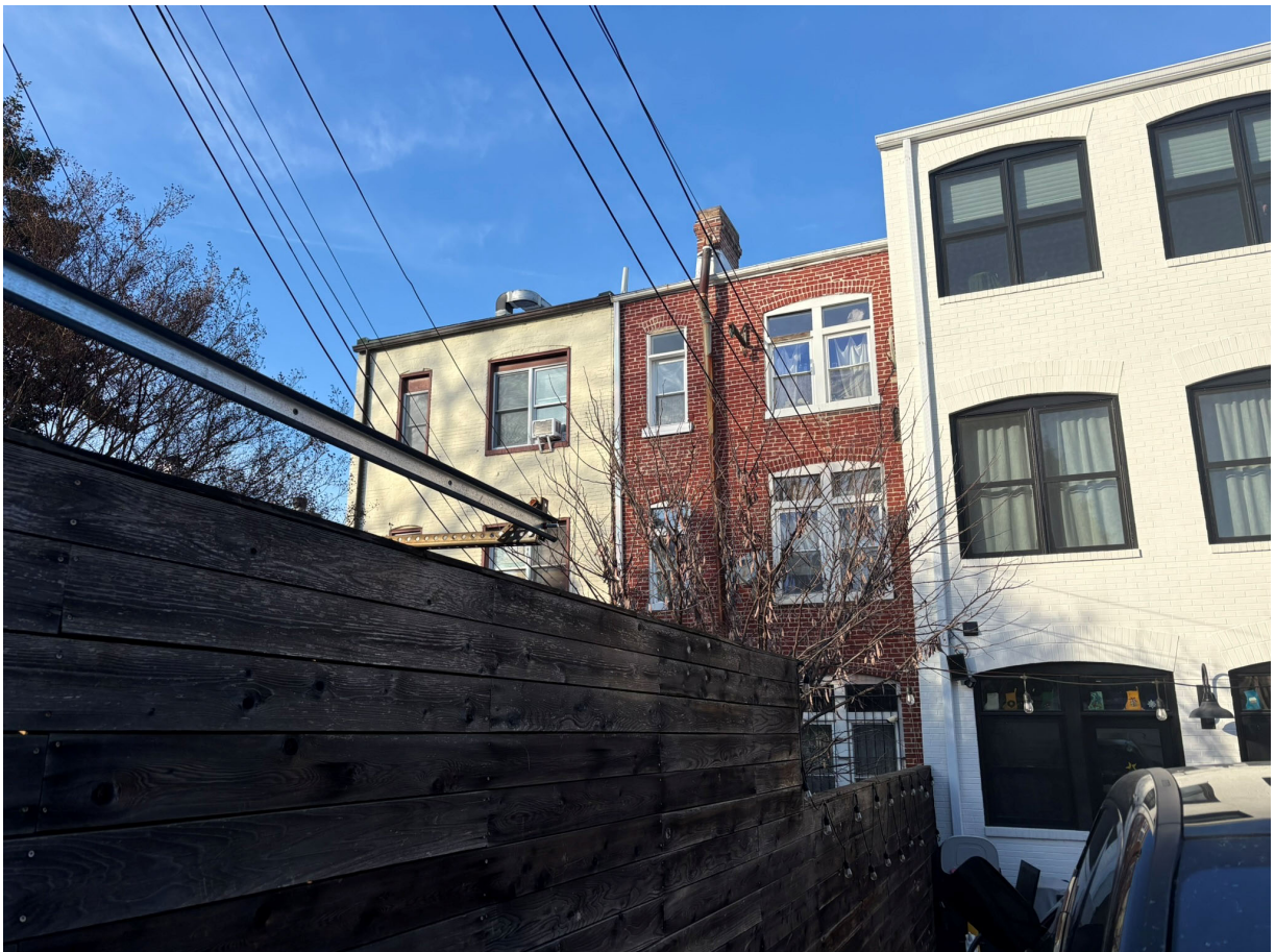
311 F STREET NE- PROPERTIES TO THE WEST
