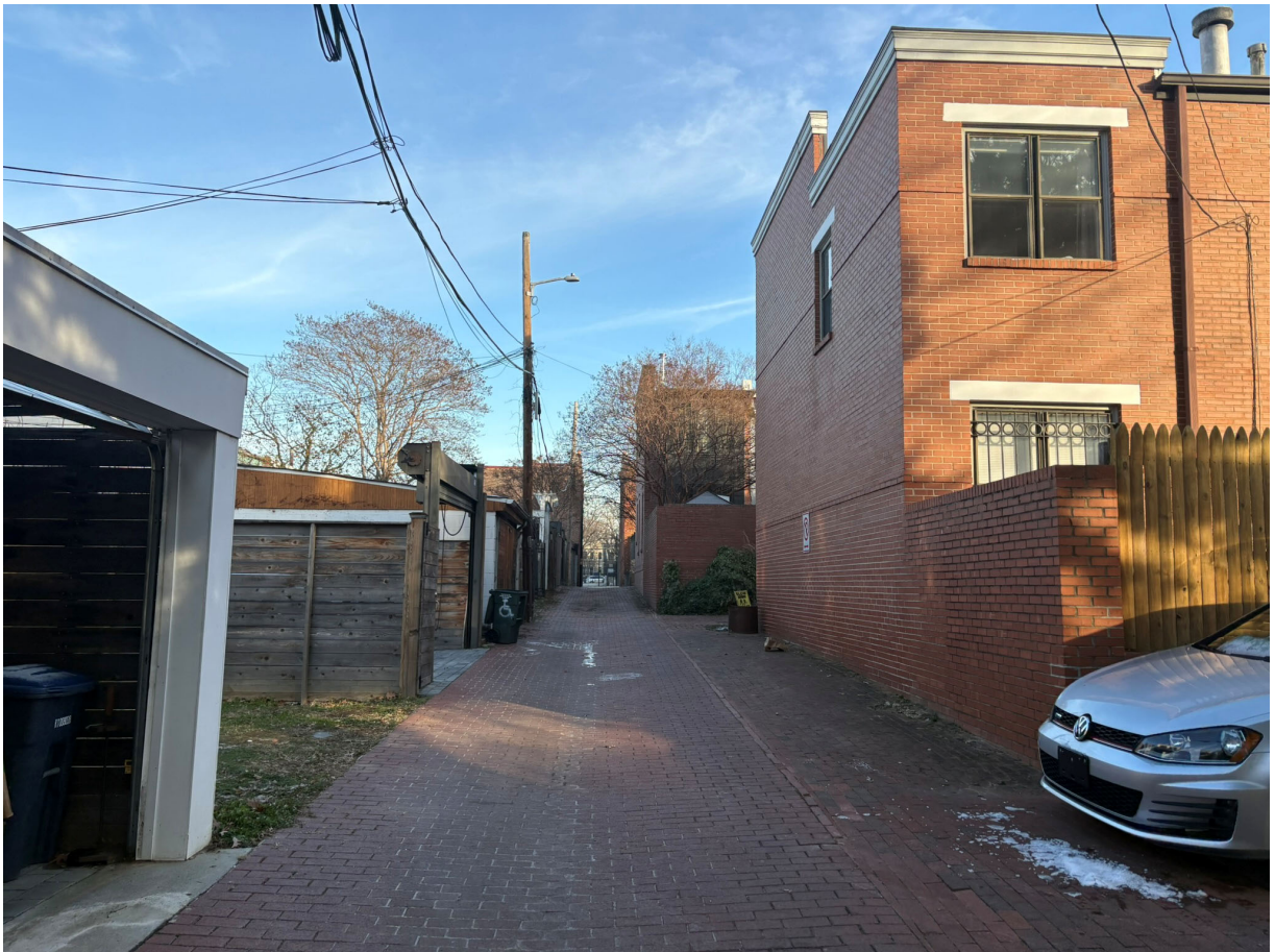
311 F STREET NE- ALLEY VIEW TO THE EAST, DWELLINGS ON GROFF COURT NE
