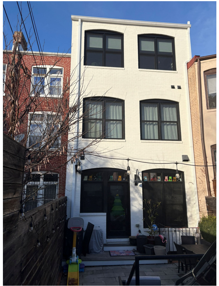
311 F STREET NE- REAR FACADE
