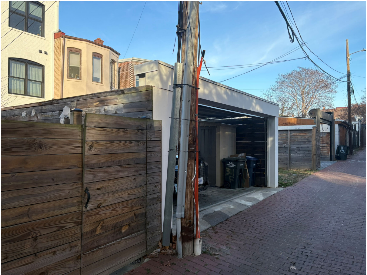
311 F STREET NE- ALLEY VIEW
