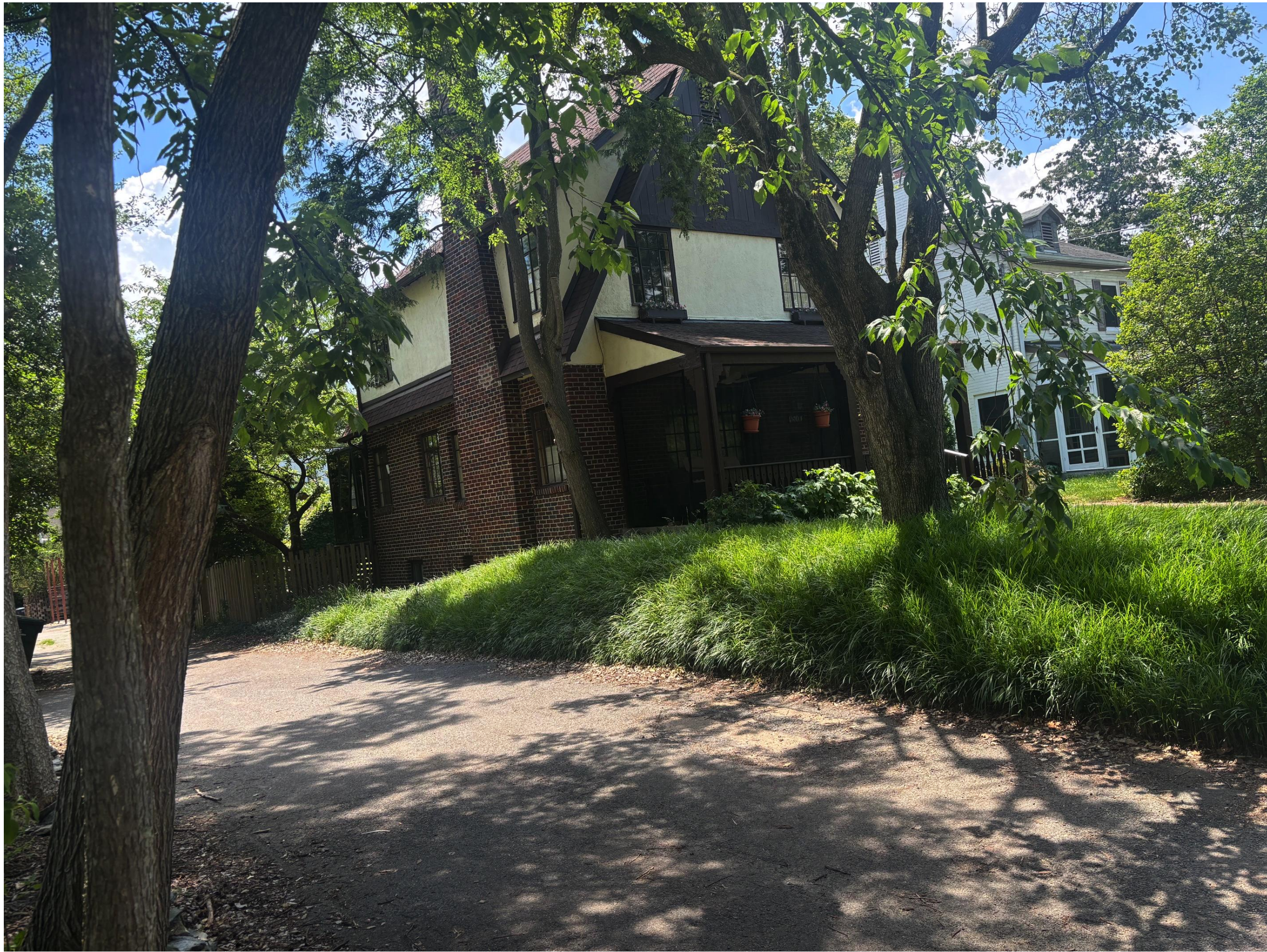
① VIEW FROM NE OF FRONT OF HOUSE
