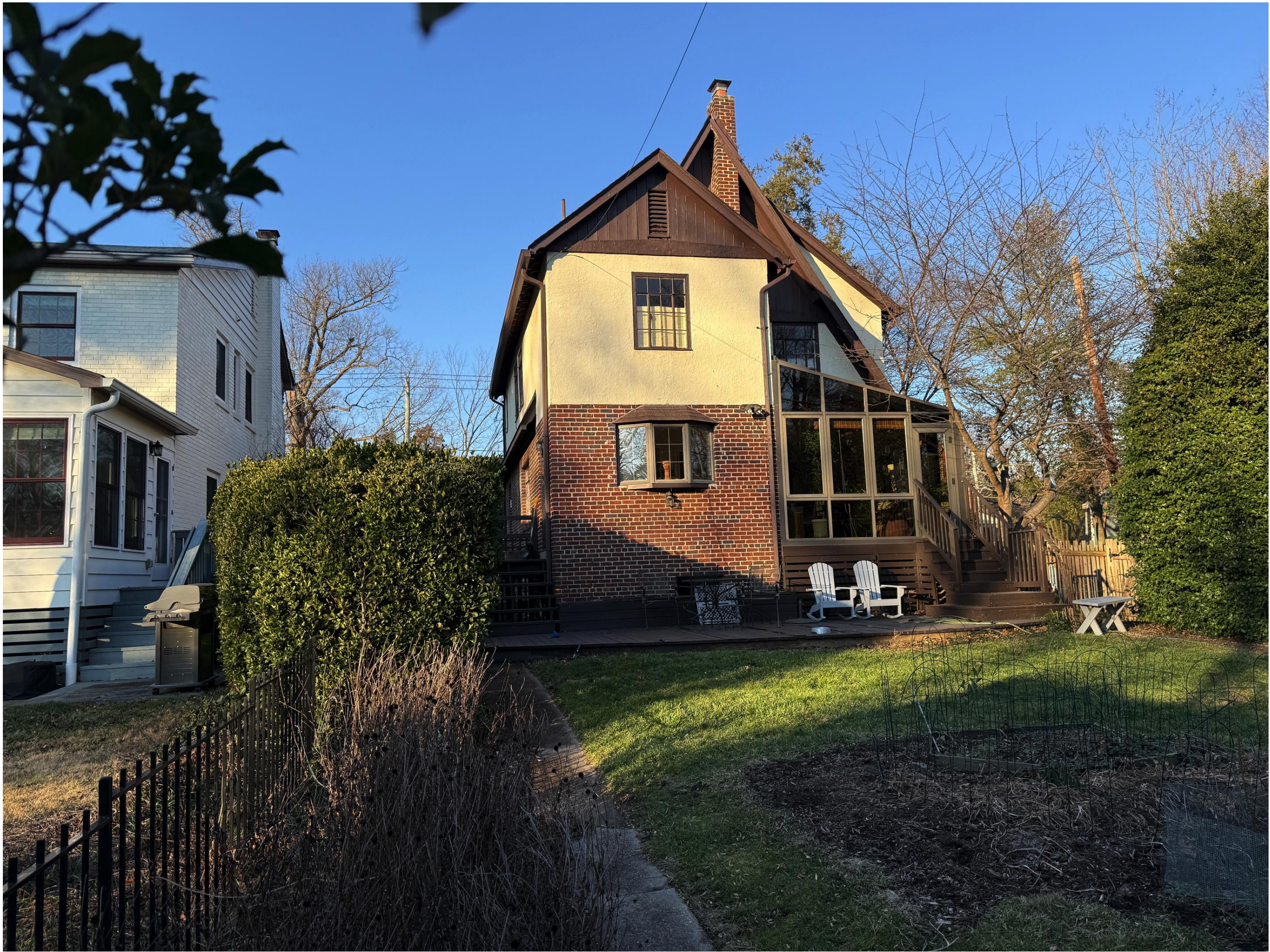
② VIEW FROM SOUTH OF REAR OF HOUSE
