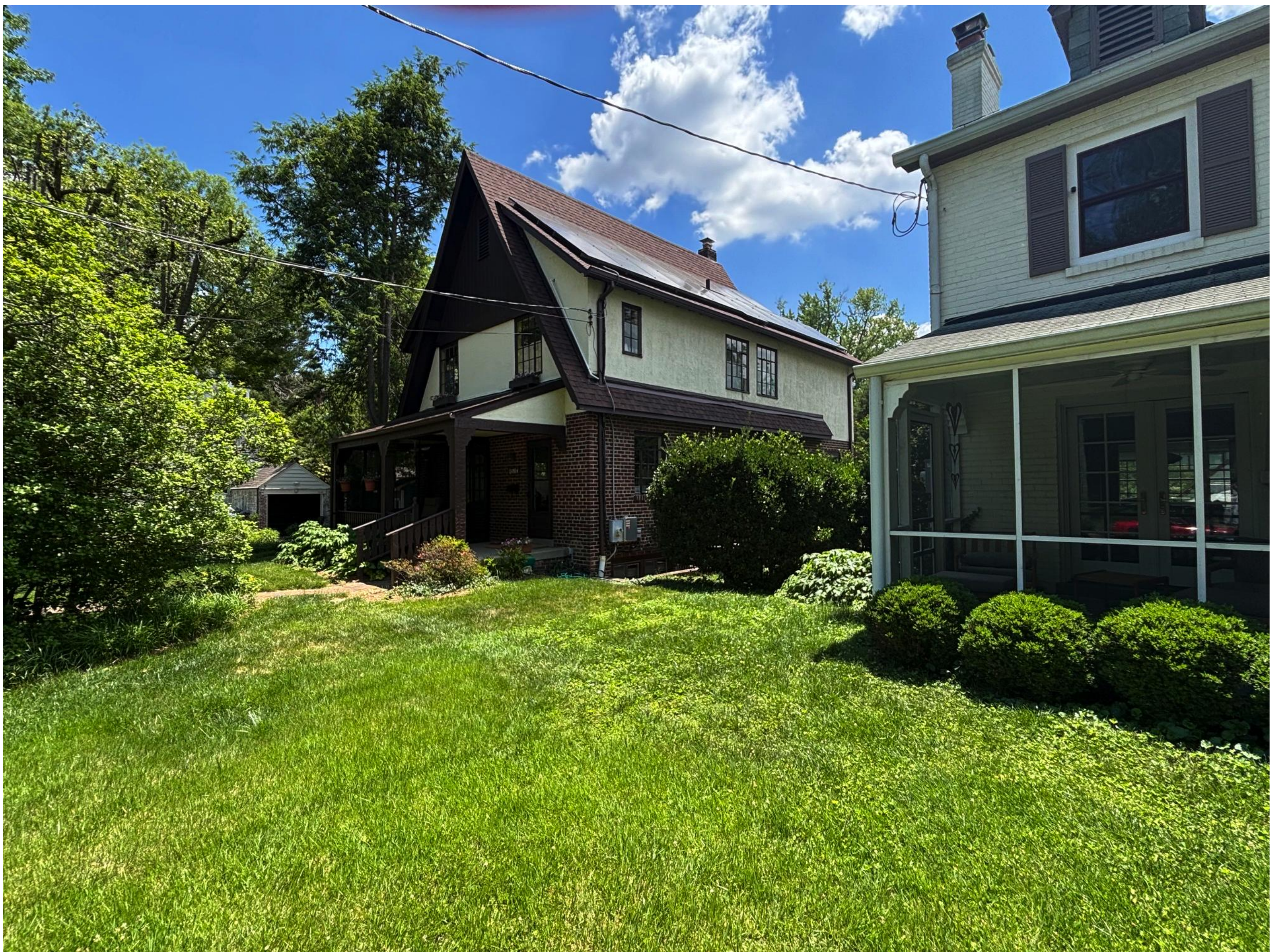
④ VIEW FROM NW OF FRONT AND SIDE OF HOUSE
