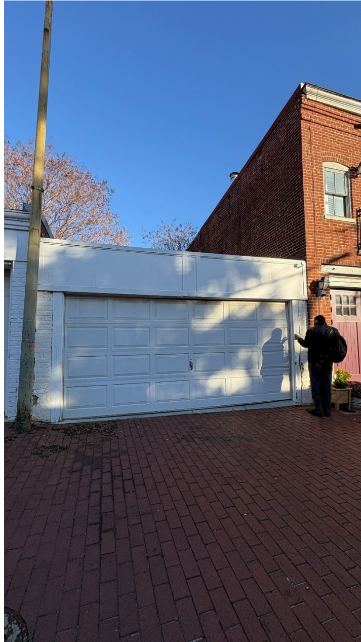
Existing Garage Alley Façade
