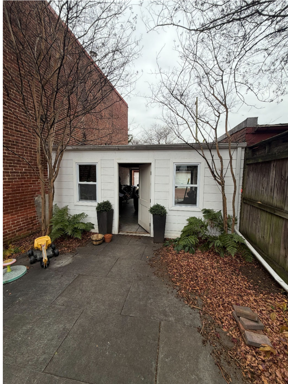
Existing Garage Yard-Facing Facade
