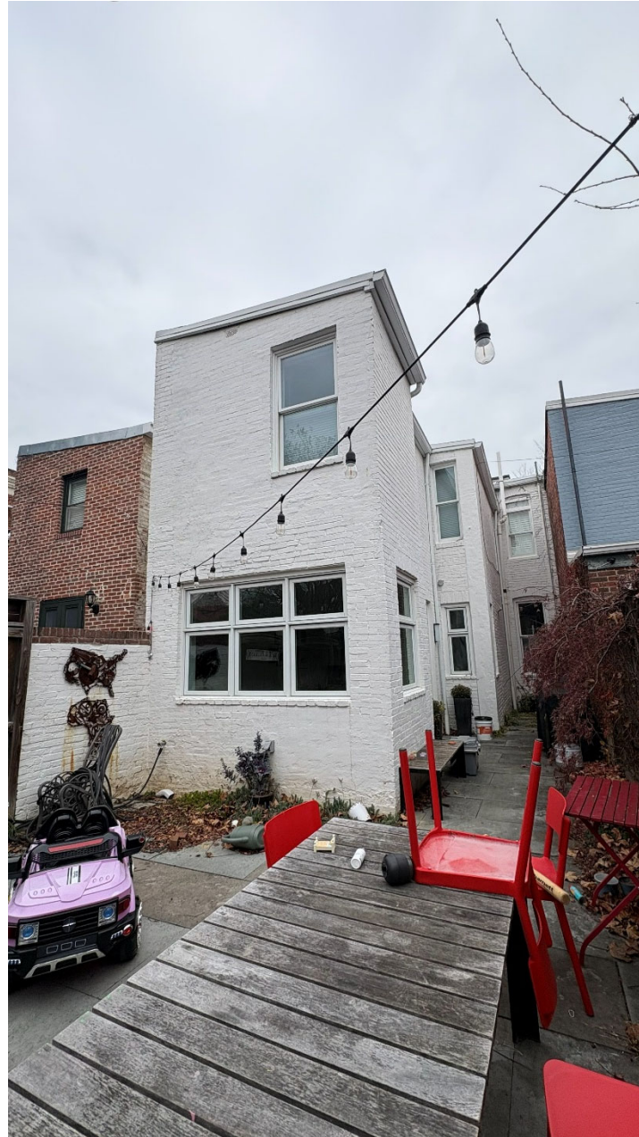
Existing House Rear Facade
