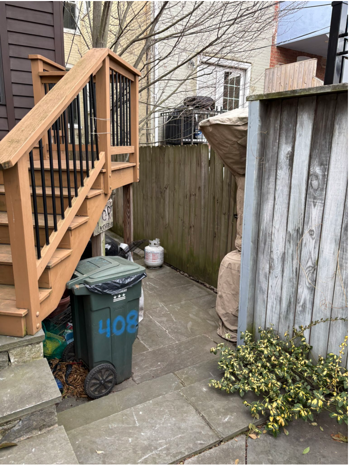
REAR FAÇADE, LOOKING WEST
