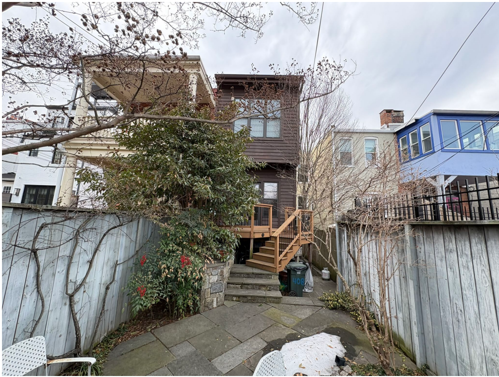
EXISTING REAR FACADE
