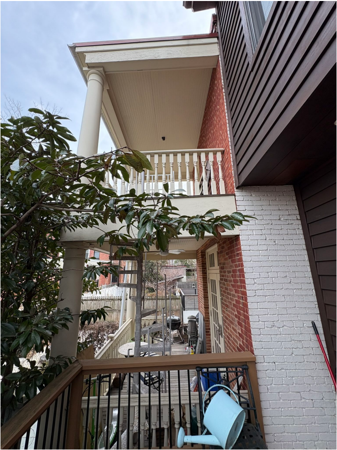
EXISTING PORCH TO EAST
