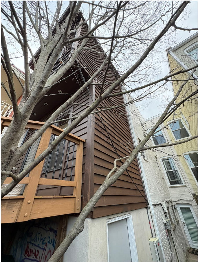
EXISTING TWO STORY REAR ADDITION
