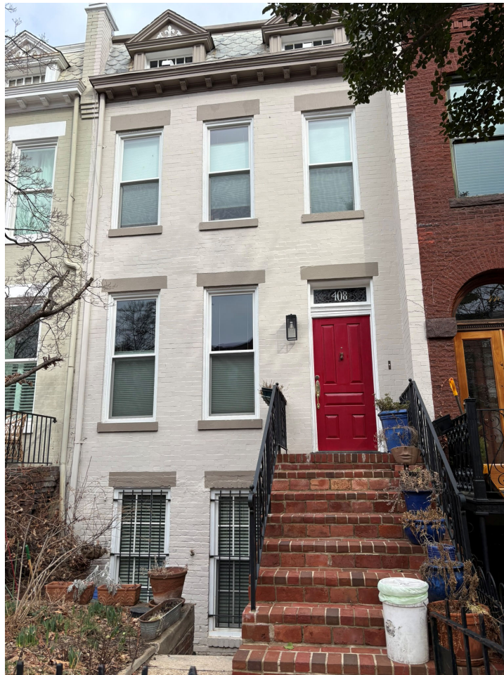
408 CONSTITUTION AVE NE- FRONT FACADE
