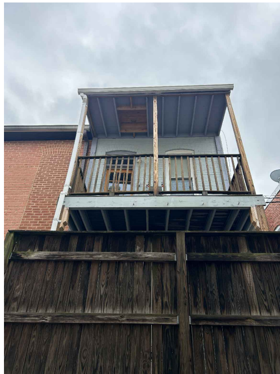
SUBJECT PROPERTY 1020 - REAR ELEVATION
