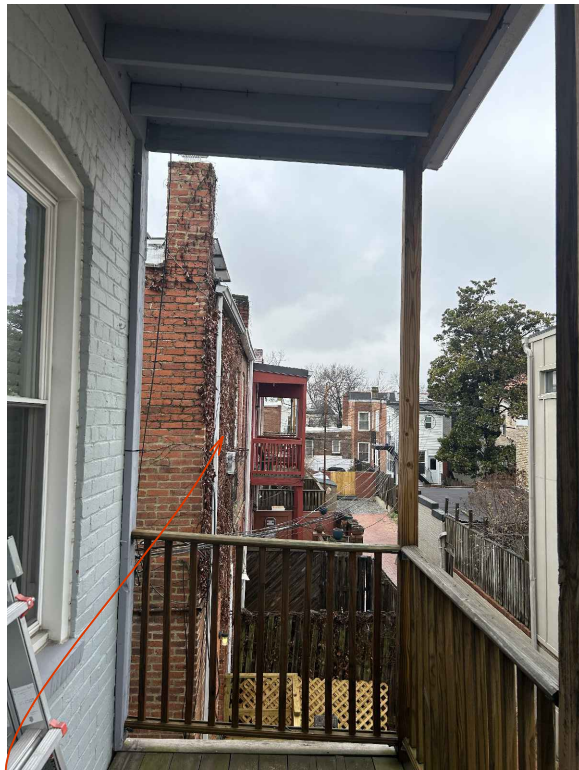
ADJACENT NEIGHBOR AT 1018 - LOOKING FROM 2ND FLOOR PORCH
