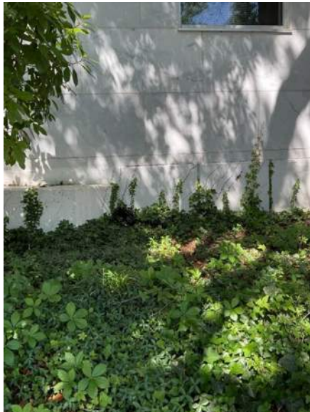
Fig. 93. Vines along the foundation of the mail room façade viewed from 25 th Street, N.W. sidewalk (LE059).
