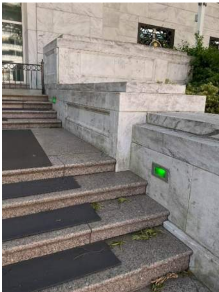
Fig. 7. Upturned anti-slip strips on stairs; green recessed lights in stairway cheek walls (LE010)
