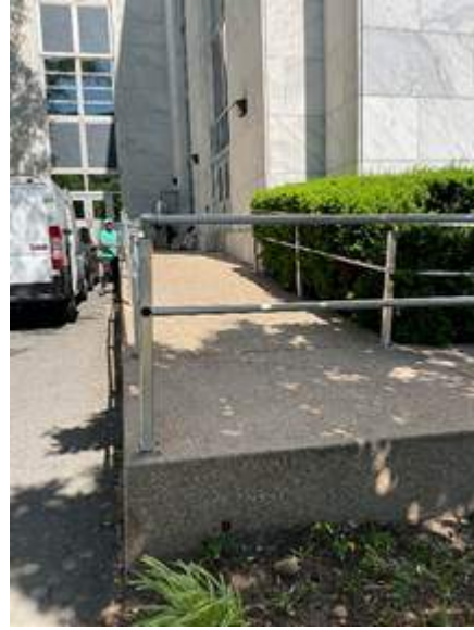
Fig. 74. Exposed aggregate ramp at the south side of the main entrance at the southeast façade (LE046).
