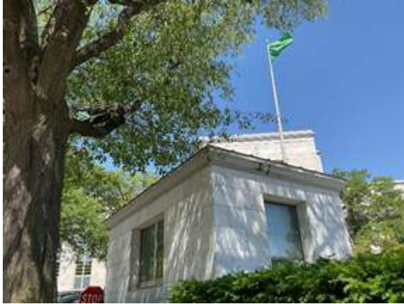
Fig. 51. View northwest from the corner of F Street, N.W., and 25 th Street, N.W. toward the mature water oak ( Quercus nigra ) south of the BCAC guard house (LE032).
