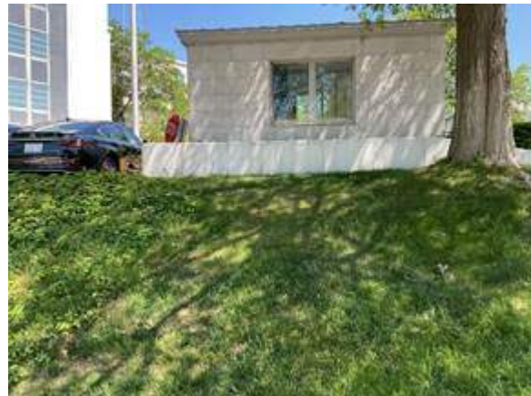
Fig. 48. View north toward the BCAC guard house from the sidewalk along F Street, N.W (LE032).
