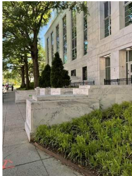
Fig. 16. View north of marble stairway at WCAC entrance; liriope groundcover at wall foundation; metal edging separating planting area from concrete sidewalk (LE010)
