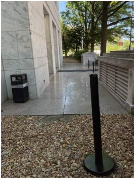
Fig. 11. View south from loose aggregate strip toward the WCAC upper landing. Ash/trash can located on the north side (LE015)
