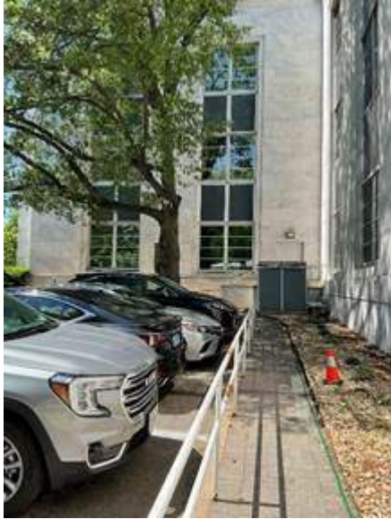
Fig. 87. View south at the parking lot along the north side of the southeast façade. The concrete paver path (LE049) leads to the shed and stairway a single door. Branches have been removed from the water oak to maintain clearance from the building.
