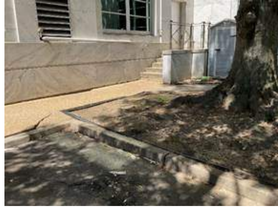
Fig. 82. Pavement at the corner of the parking lot, north of the southeast façade main entrance. Stairs lead to a door at the north side of this façade (LE048).
