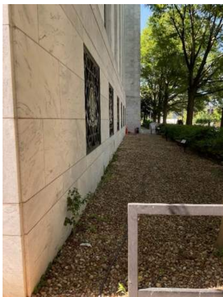
Fig. 105. View southwest along the southwest façade of the Embassy (New Hampshire Avenue, N.W.) from the northern corner of the building. Access to the aggregate foundation area is blocked by a metal fence (LE071, LE011).
