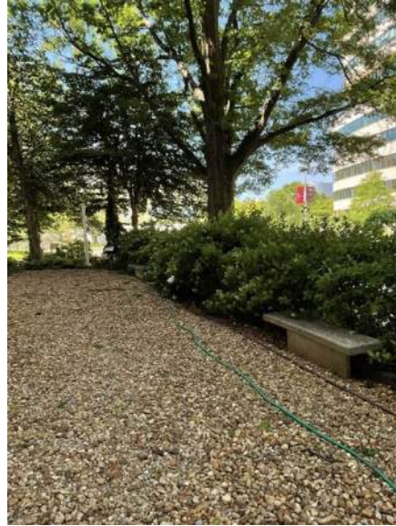
Fig. 14. View south of loose aggregate strip at foundation - two concrete benches situated along the euonymus shrub border (LE011 & LE012)
