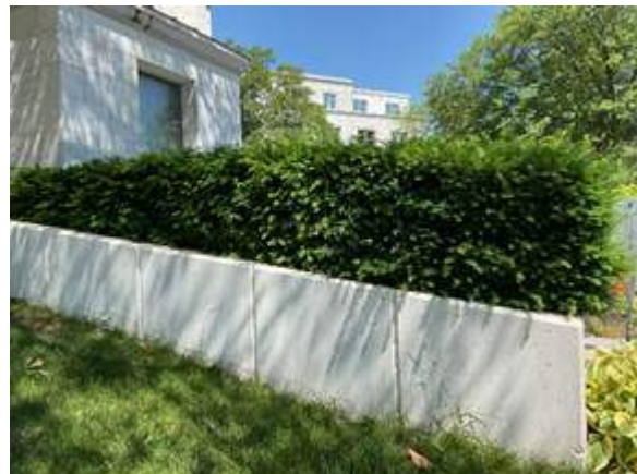
Fig. 50. View northwest toward the guard house. White concrete wall following the slope of the terrain and retaining a row of evergreen yews (LE041).
