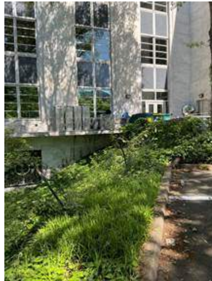
Fig. 72. Sloping terrain south of the parking lot, near the dumpster, with a dilapidated wire fence along the perimeter (LE056).
