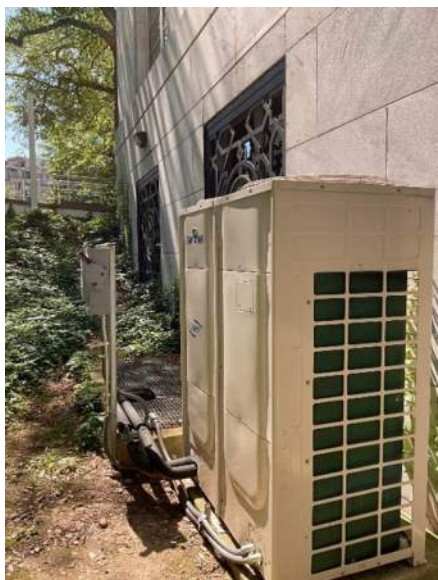
Fig. 109. A/C unit and window well at the north façade of the Embassy (LE076).
