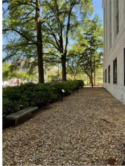
Fig. 10. View north of loose aggregate strip at foundation – three concrete benches situated among the euonymus shrub border (LE011 & LE012)
