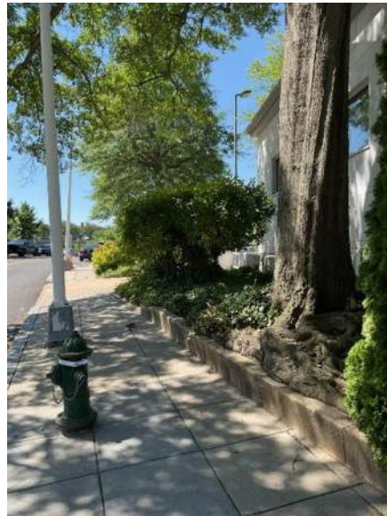
Fig. 94. View south along 25 th Street, N.W., east of the mail room. A concrete curb defines the planting area border. Roots of the water oak engulf the concrete curb (LE060).
