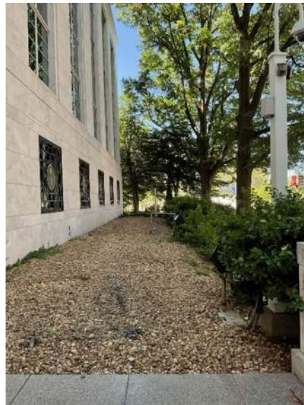
Fig. 12. View north to loose aggregate strip south of WCAC entrance stairway landing (LE011)
