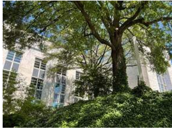
Fig. 46. View toward the southeast façade from the public sidewalk. Water oak trees ( Quercus nigra ) provide shade. Invasive English ivy spreads into the trees and forms an unruly mass at the base (LE040).
