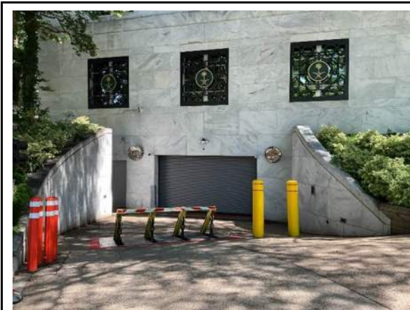
Fig. 23. PCAC Garage entrance with separate doors for vehicles and staff; sloping marble retaining walls (LE021)
