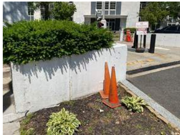
Fig. 54. Concrete wall north of the pedestrian access stairway, and south of the BCAC vehicle screening area (LE041).
