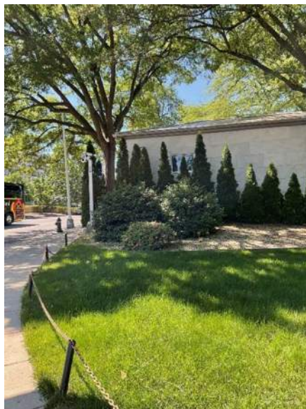
Fig. 96. View south on 25 th Street, N.W., toward the mail room. 76 cm (30 in) diameter water oak is at the building corner. Conical arborvitae, hollies, and blooming azalea compose the foundation planting. Turf grass and a single chain fence meet the public sidewalk (LE059-67).
