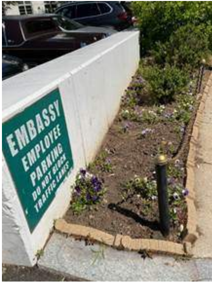
Fig. 57. Concrete wall north of the BCAC vehicle screening area with Embassy Employee Parking sign. Seasonal color (pansies) and bare soil are bordered with concrete unit edging stones and low, single chain barrier (LE044).
