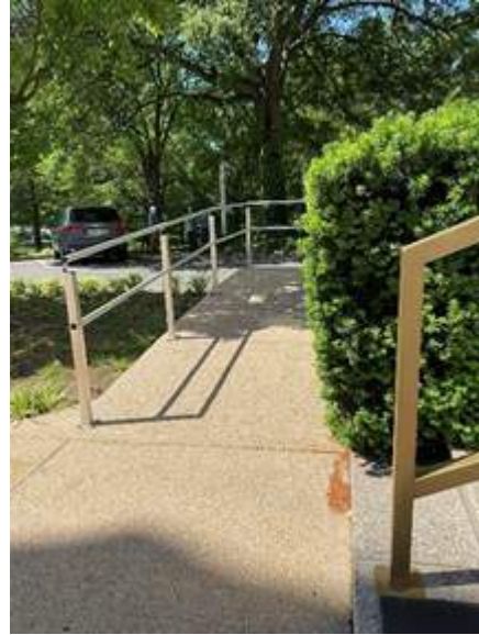
Fig. 78. Exposed aggregate ramp to the south of the main entrance at the southeast façade (LE046, LE045). The stair handrail and yew foundation plantings are pictured at right. Parking and mature water oaks are in the background.
