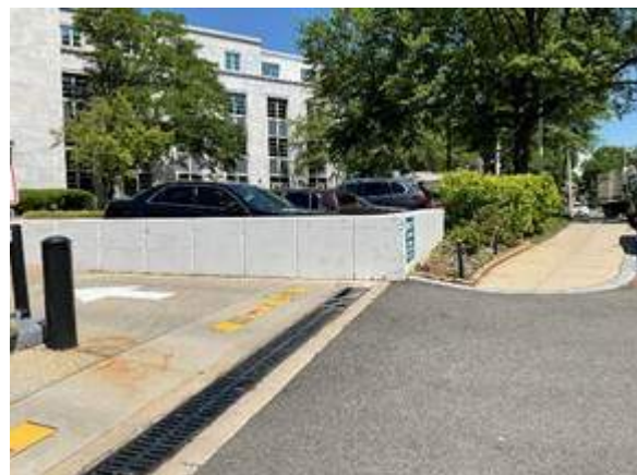
Fig. 56. View northwest to the southeast façade and concrete wall to the north of the BCAC vehicle screening area. View of the public sidewalk along 25 th Street, N.W., at right (LE044).
