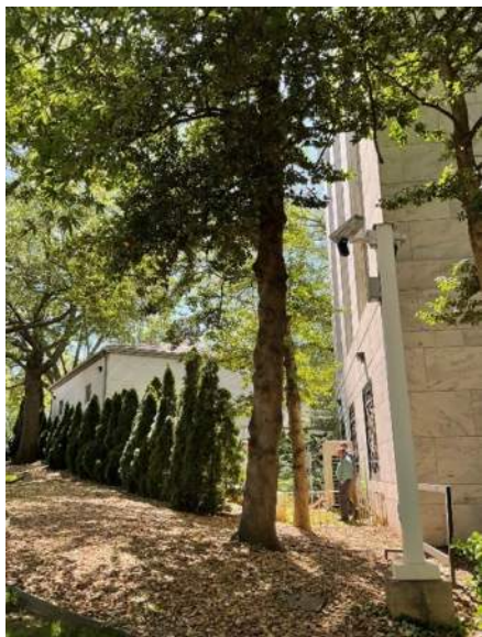
Fig. 103. View east toward the west façade of the mail room and north façade of the Embassy, from the public sidewalk. Row of conical arborvitae shrubs descends the terrain to a mature, limbed up holly tree. A/C unit pictured at the foundation of the Embassy (LE071).
