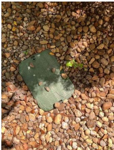
Fig. 107. Irrigation control valve box in the loose aggregate surface at the north corner of the Embassy (LE073).
