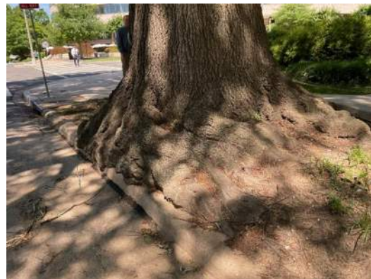
Fig. 30. View west along F Street N.W. Roots of the 3.8 m circumference willow oak tree envelop the curb along F Street, N.W. (LE018)
