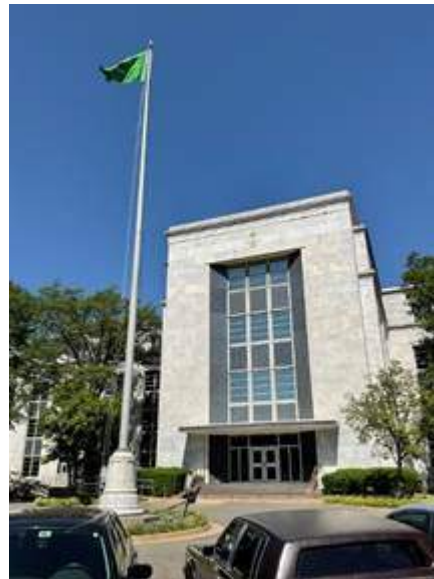
Fig. 68. View northwest to the southeastern façade main entrance (from the public sidewalk on 25 th Street, N.W.) flanked by small magnolia trees in the front and mature water oaks at the sides (LE043, LE042).
