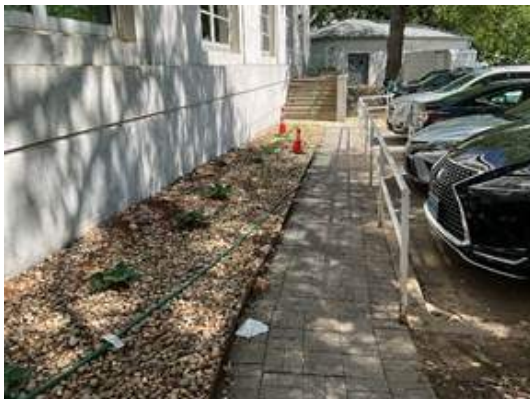
Fig. 85. Parking along the southeast façade is separated from the narrow paver walkway by a white metal railing (LE052). The paver surface is uneven and likely upended by nearby oak roots (LE049). MCAC building and stairs to two separate doorways pictured in the background (LE053).
