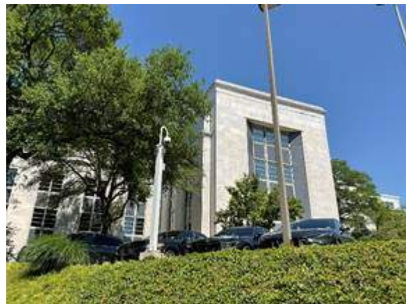
Fig. 42. View up toward the east façade from the public sidewalk on F Street, N.W. Mature water oaks are located to the north and south of the entrance (LE040).
