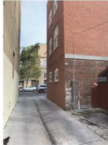
9. Alley Entrance from 5th Street NW
