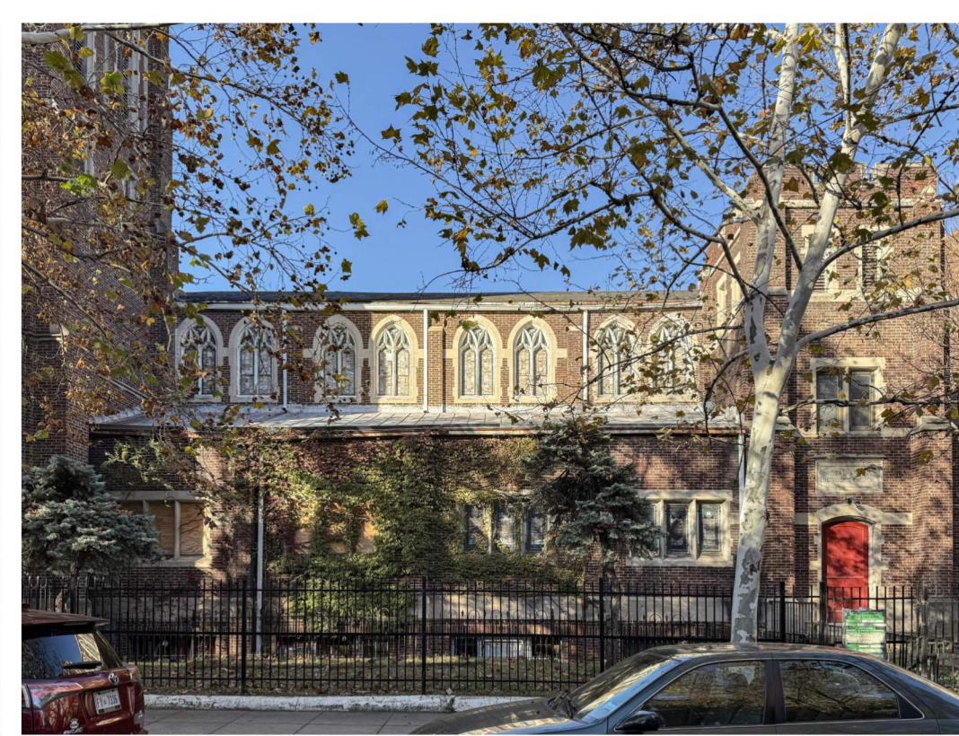
3. COLUMBIA RD NW - VIEW OF 1914 ADDITION
