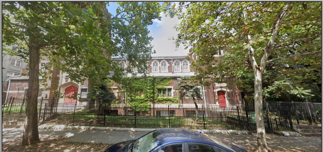
View from Columbia Road, NW directly facing the Property:
