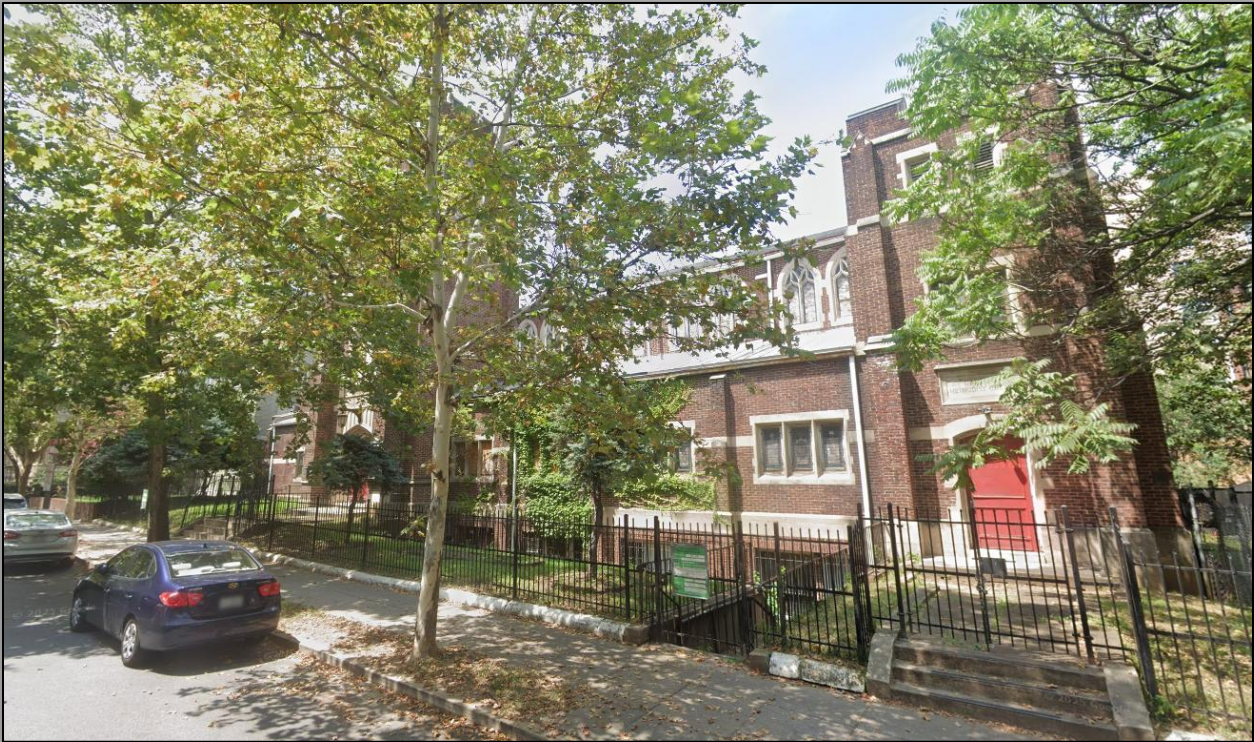
View from Columbia Road, NW facing west:
