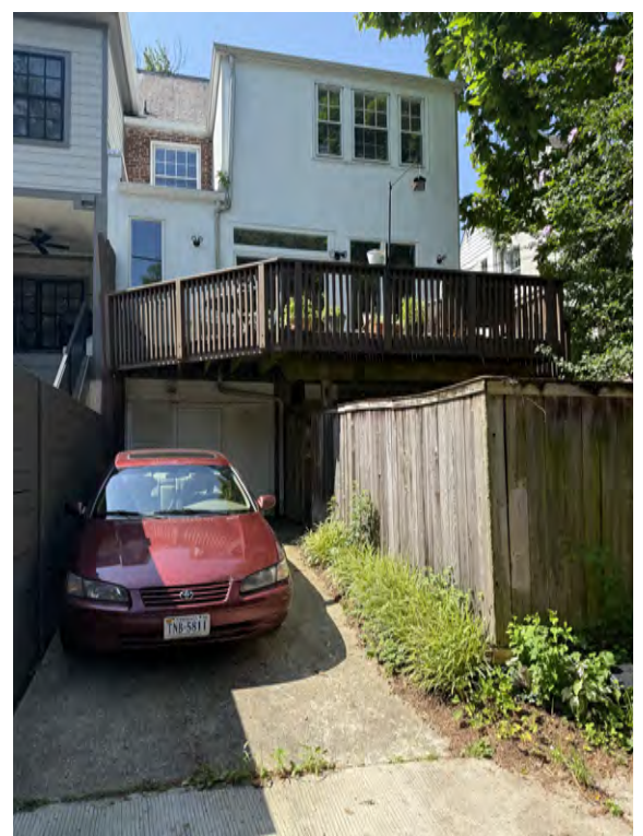
PHOTO OF EXISTING DECK AT LOT 36
