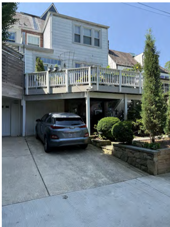
PHOTO OF EXISTING DECK AT LOT 38
