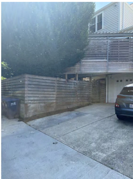
PHOTO OF EXISTING DECK AT LOT 37
