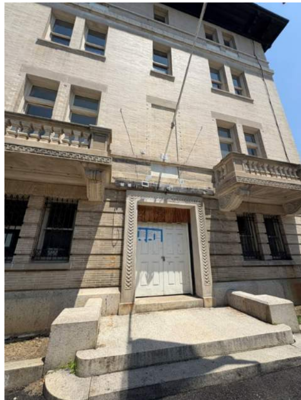
EXISTING ENTRY CONDITION
