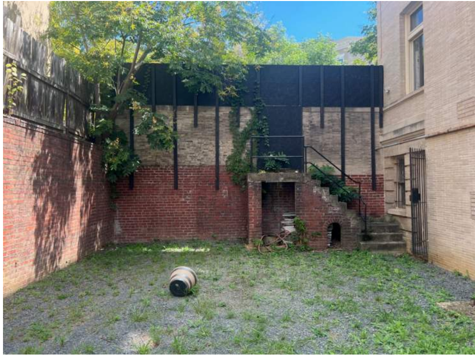
FACING EAST TOWARD RETAINING WALL AGAINST 22ND STREET, NW
