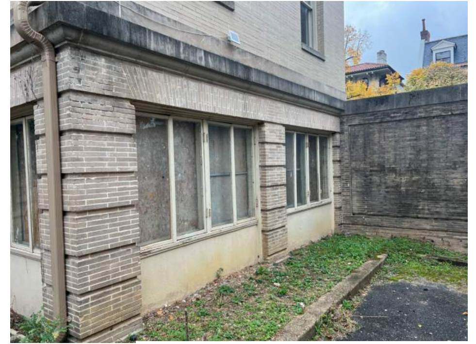
AREA OF PROPOSED GARAGE DOORS
