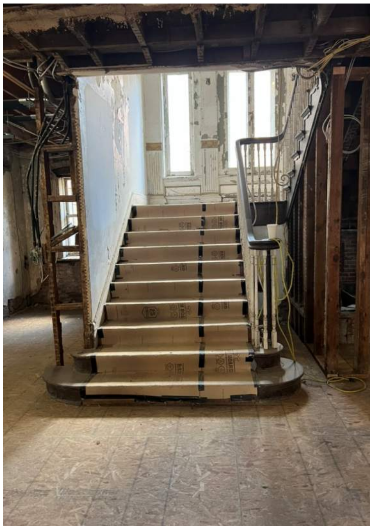
STAIR AT 1ST FLOOR
