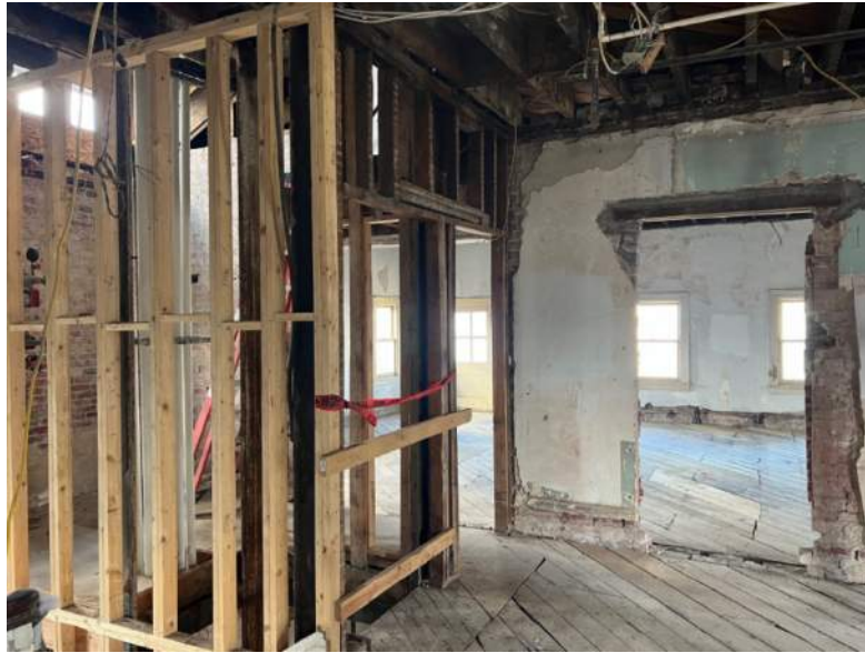
3RD FLOOR STAIR HALL FACING NORTH
