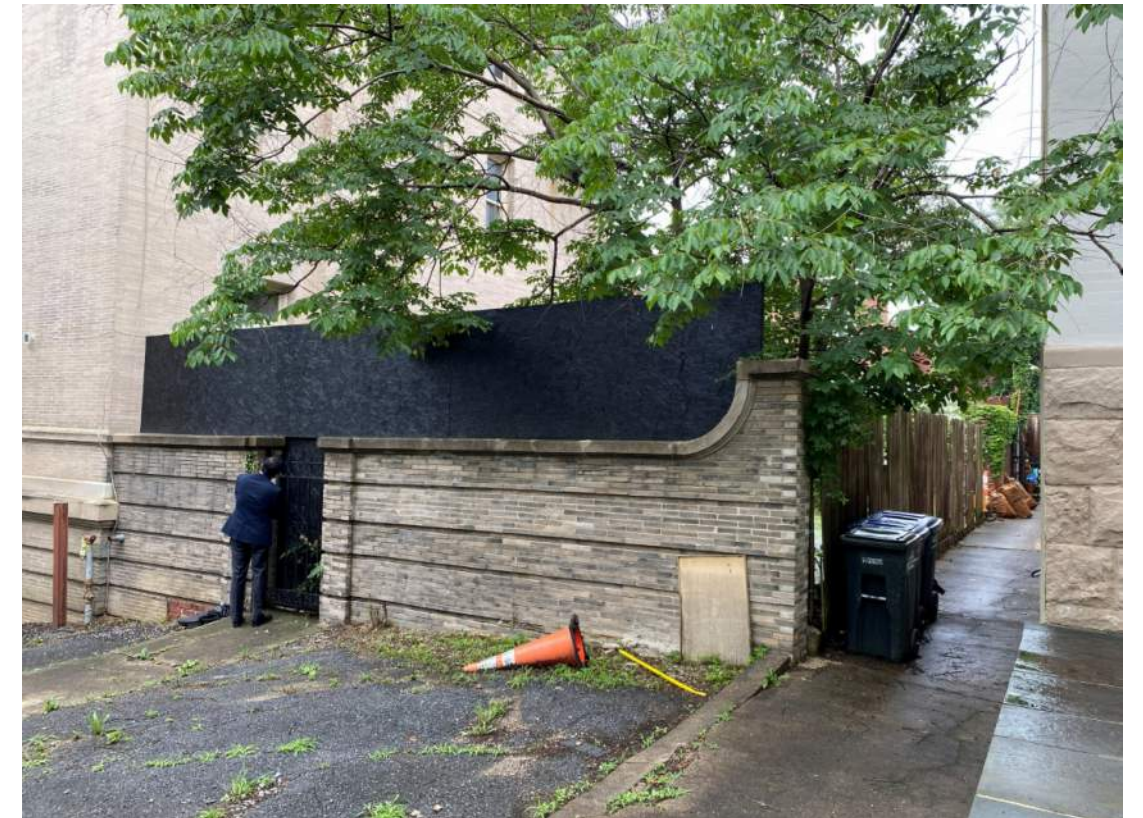
GATE FACING 22ND STREET, NW
