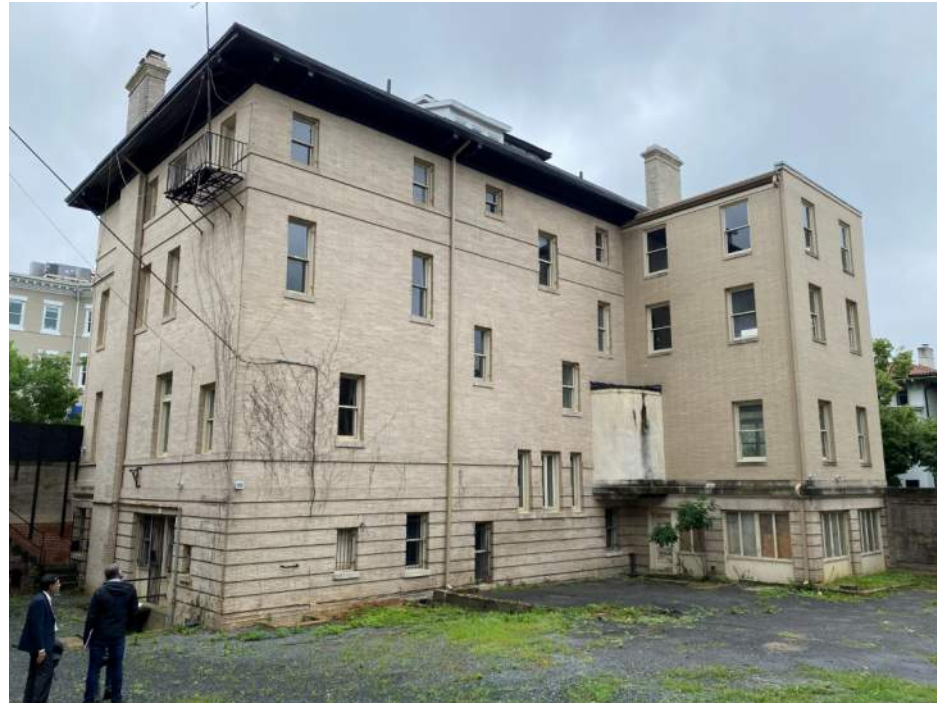
INSIDE CORNER AND PROPOSED LOCATION FOR NEW STAIR
