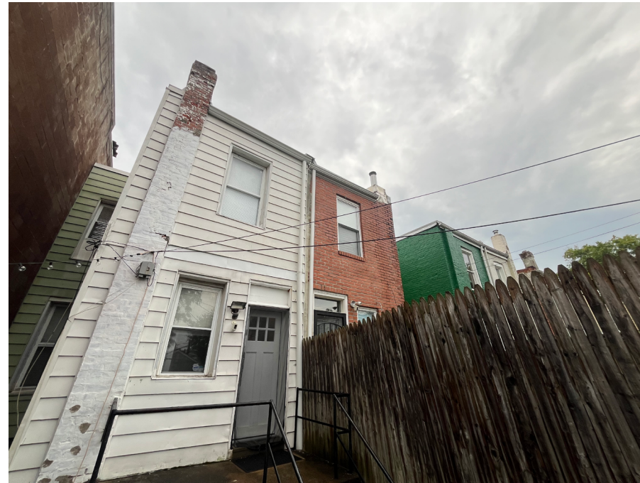
4. VIEW LOOKING SE FROM REAR YARD OF 443 17TH ST SE
