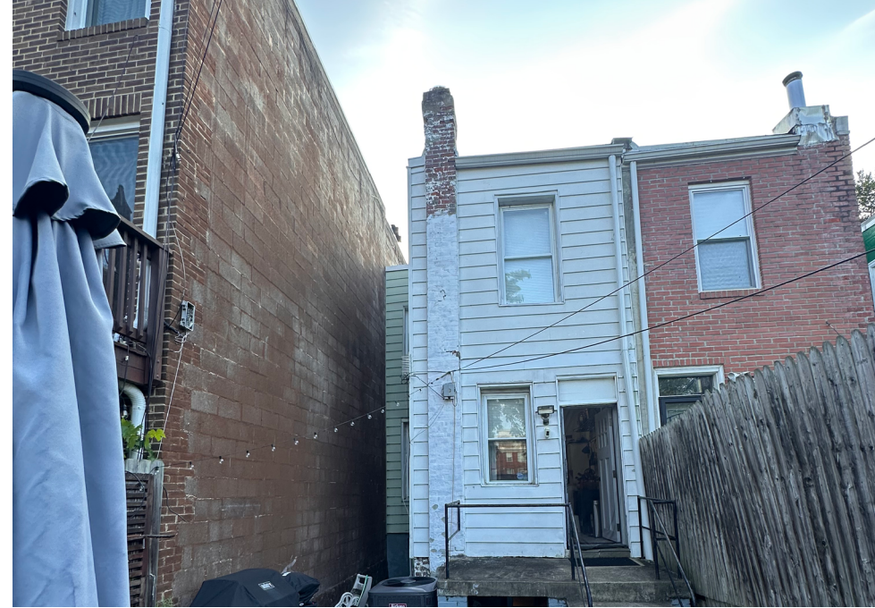
6. VIEW LOOKING E FROM REAR YARD OF 443 17TH ST SE
