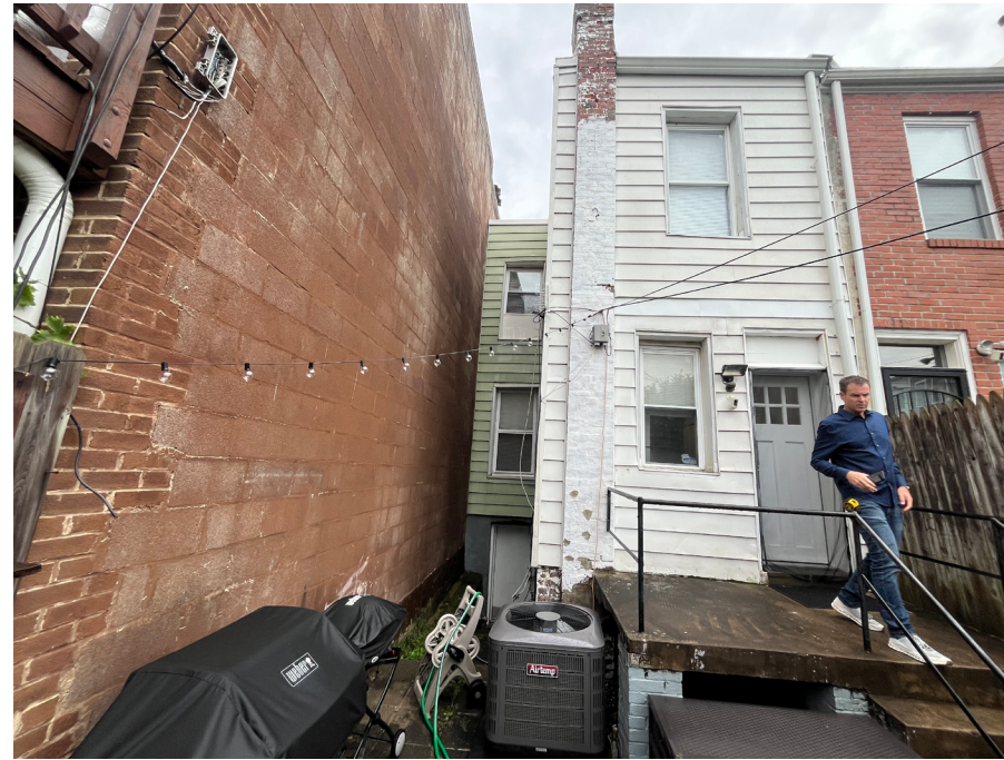
2. VIEW LOOKING E FROM REAR YARD OF 443 17TH ST SE
