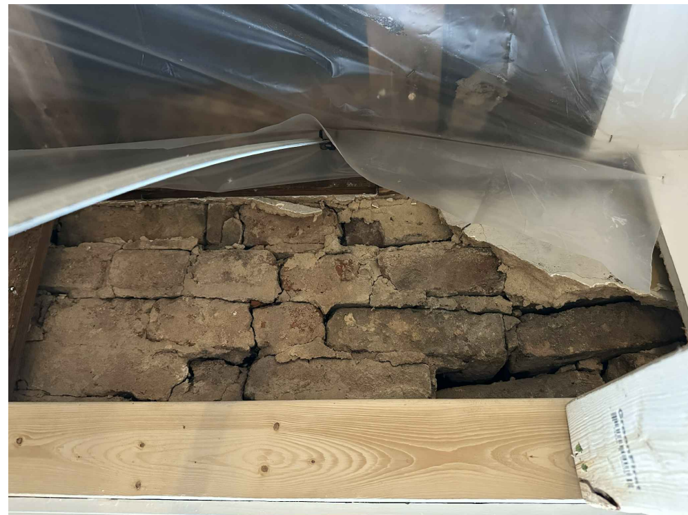
DAMAGED BRICK
