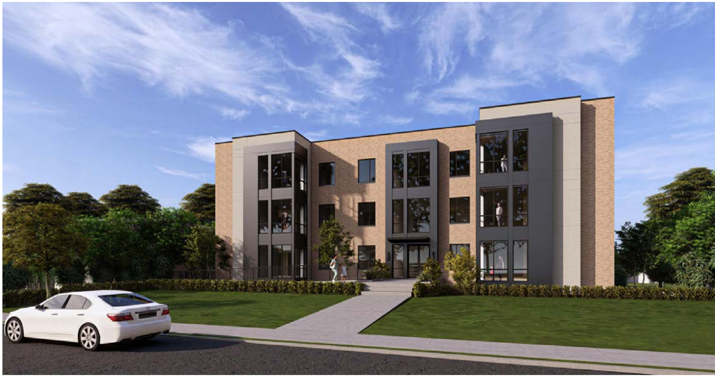
FRONT VIEW ACROSS ALABAMA AVE
