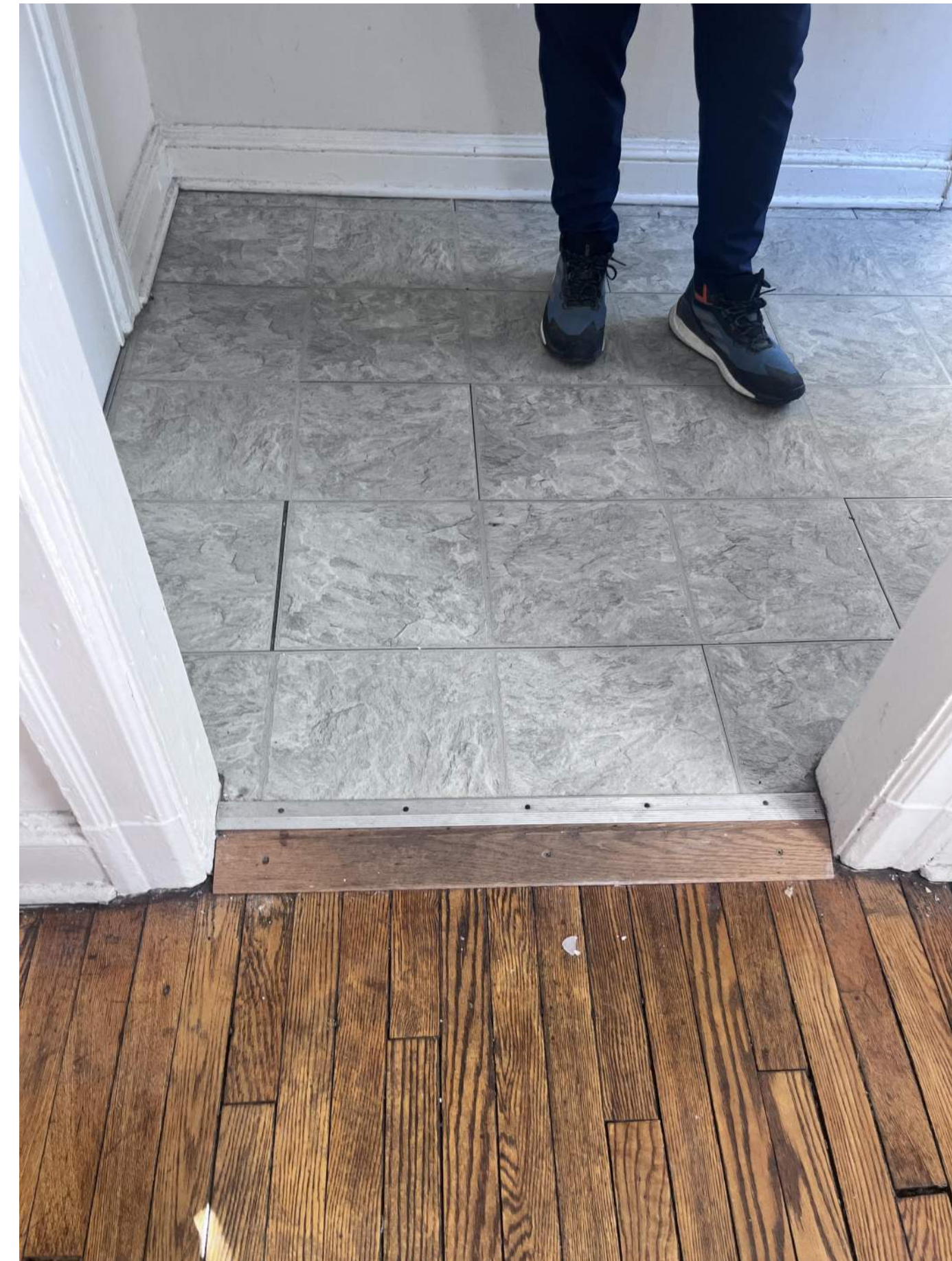
3. REPAIR & REPLACE DAMAGED FINISHES THROUGHOUT
