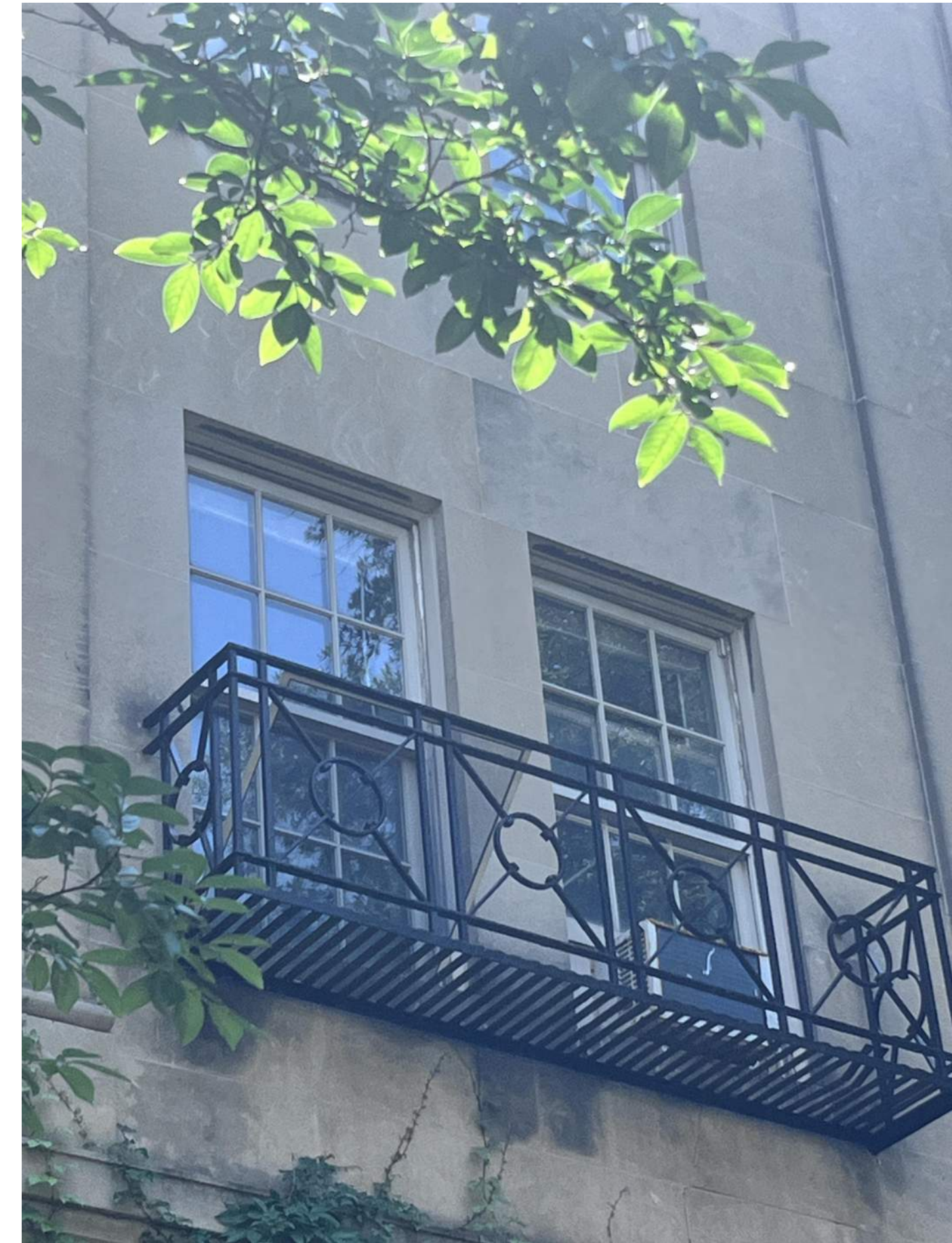
2. LIMESTONE CLEANING AND REPAIR HISTORIC FACADE
