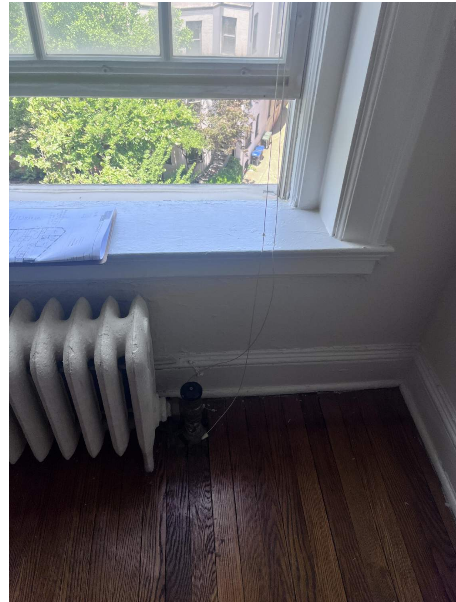
7. REPLACE OUTDATED HVAC SYSTEM UPGRADE TO MEET CODE, WINDOW REPLACEMENT WITH ENERGY EFFICIENT WINDOW
