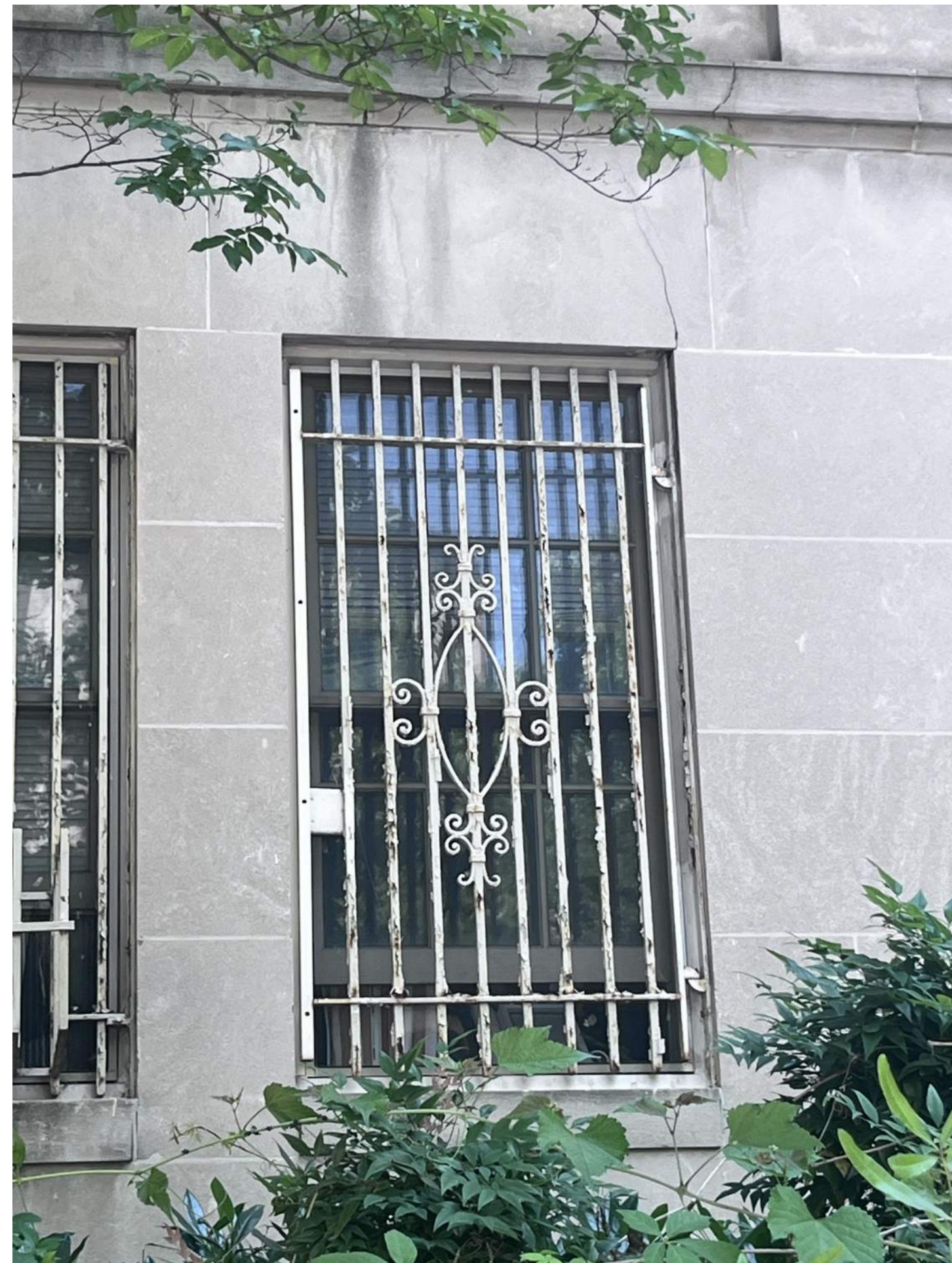
6. REMOVE RUSTED SECURITY GRILL FROM WINDOWS, REPAIR CRACKS IN STONE FACADE
