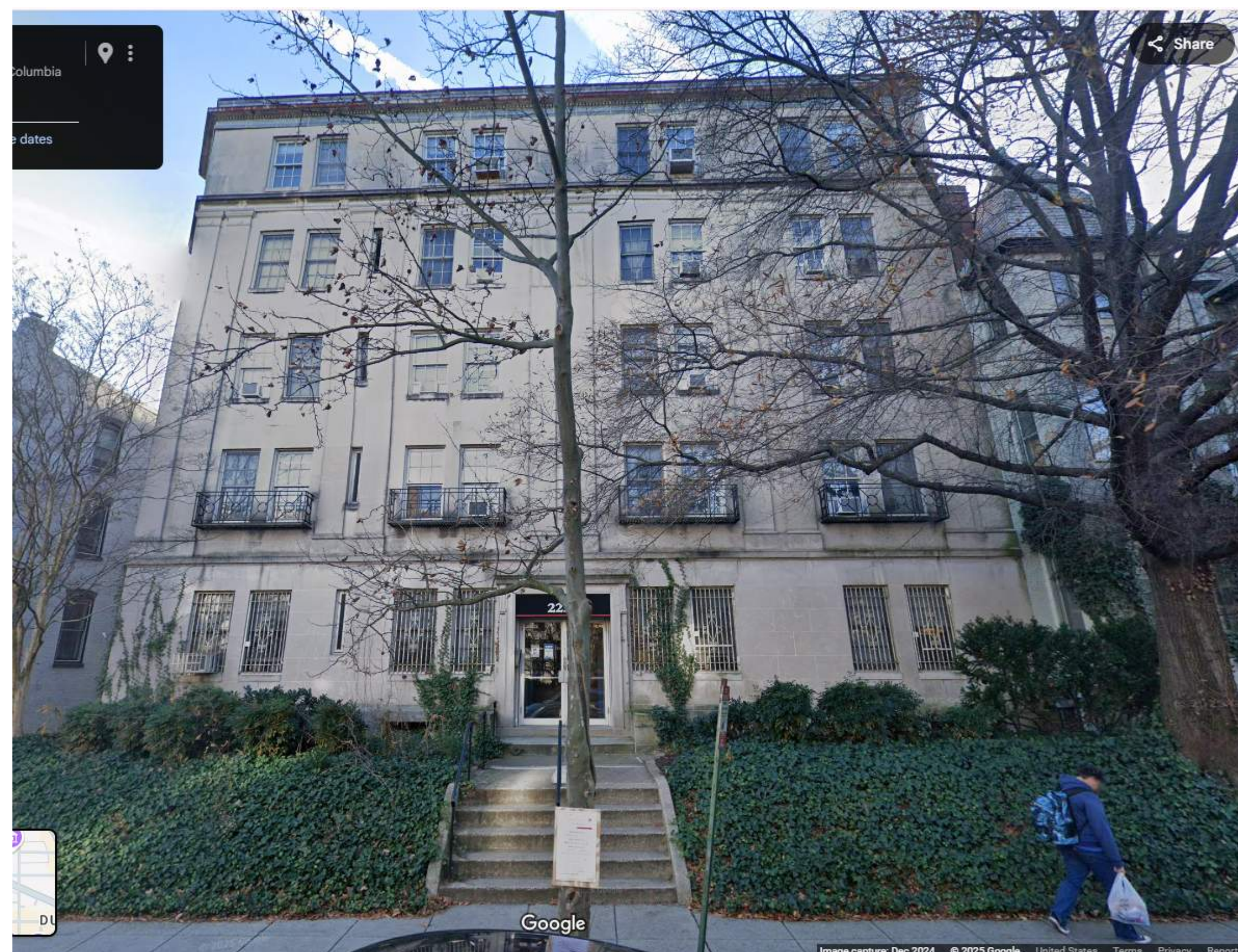
2. VIEW OF Q ST. FACADE (NORTH)
