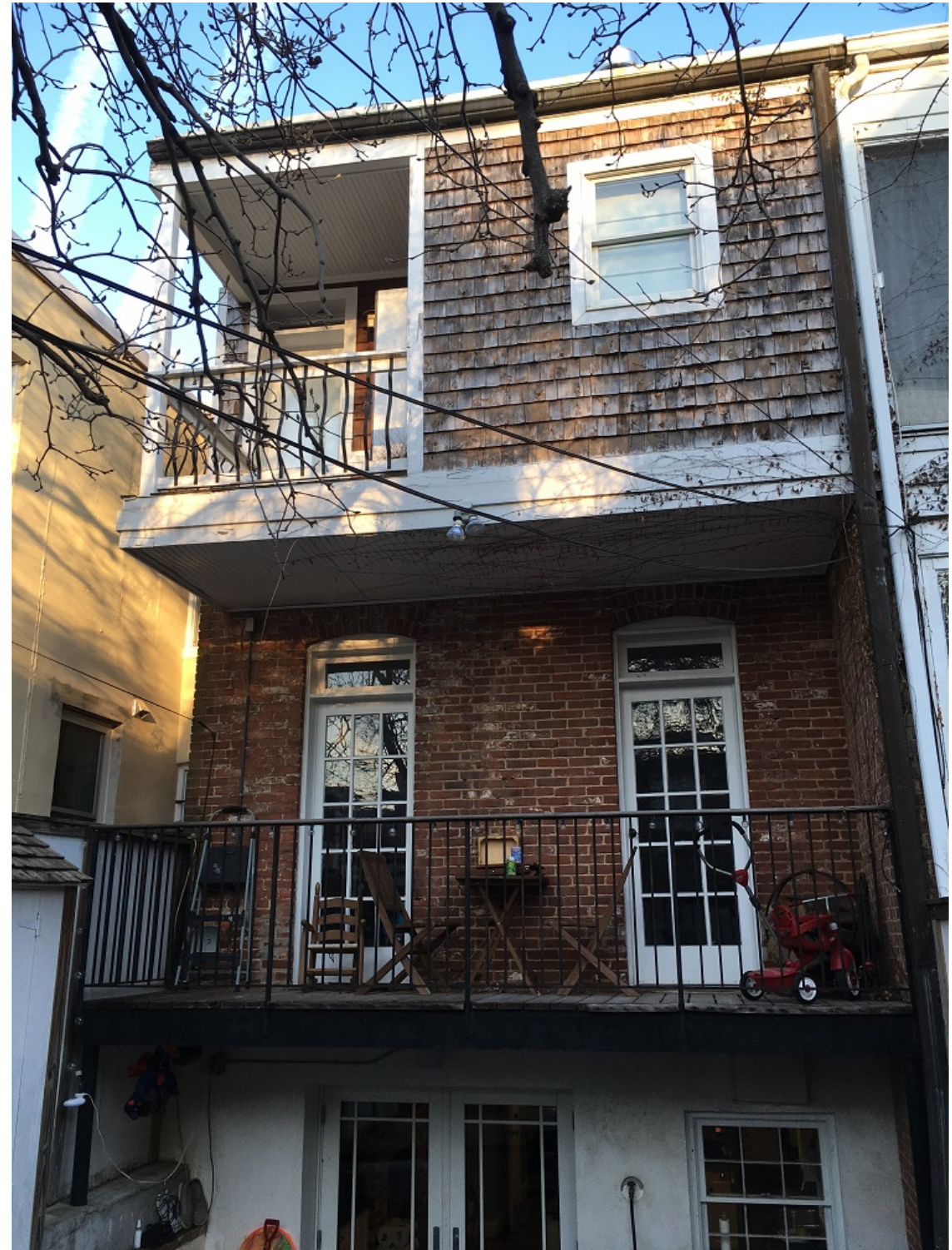
EXISTING REAR FAÇADE
