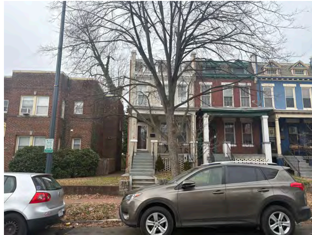
VIEW ACROSS 5 TH STREET NE
