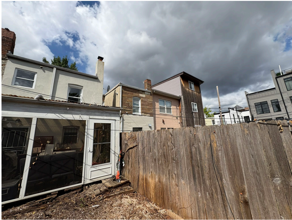
REAR VIEW LOOKING NORTH
