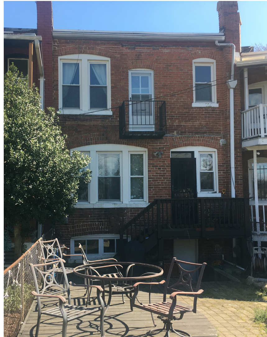
130 Rhode Island Avenue NE Rear Yard of Site
