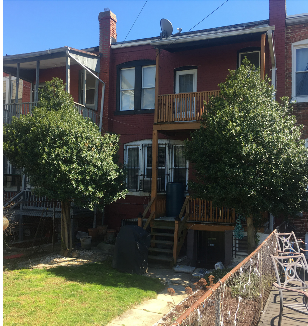
132 Rhode Island Avenue NE Eastern Adjoining Rowhouse
