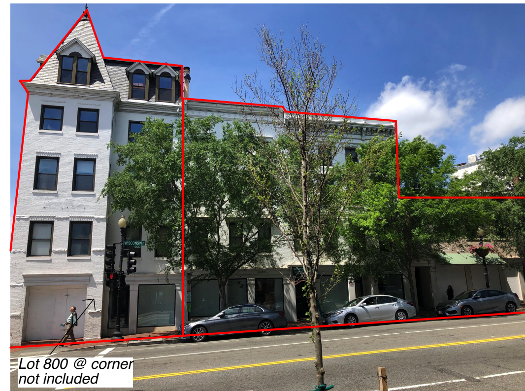
2. View from Wisconsin Ave
