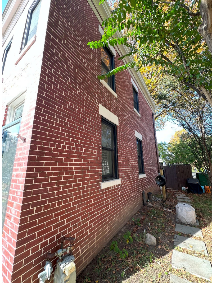
14 th St. Street Facade
