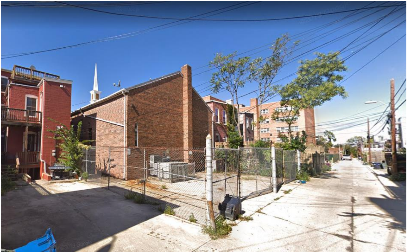
View of 3423 Holmead Place, N.W. from the rear alley.
