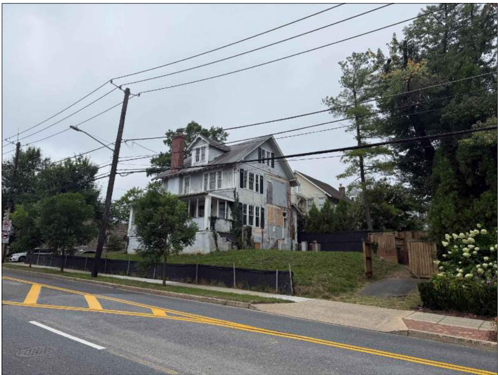
RIGHT SIDE WITH EXISTING DRIVEWAY
