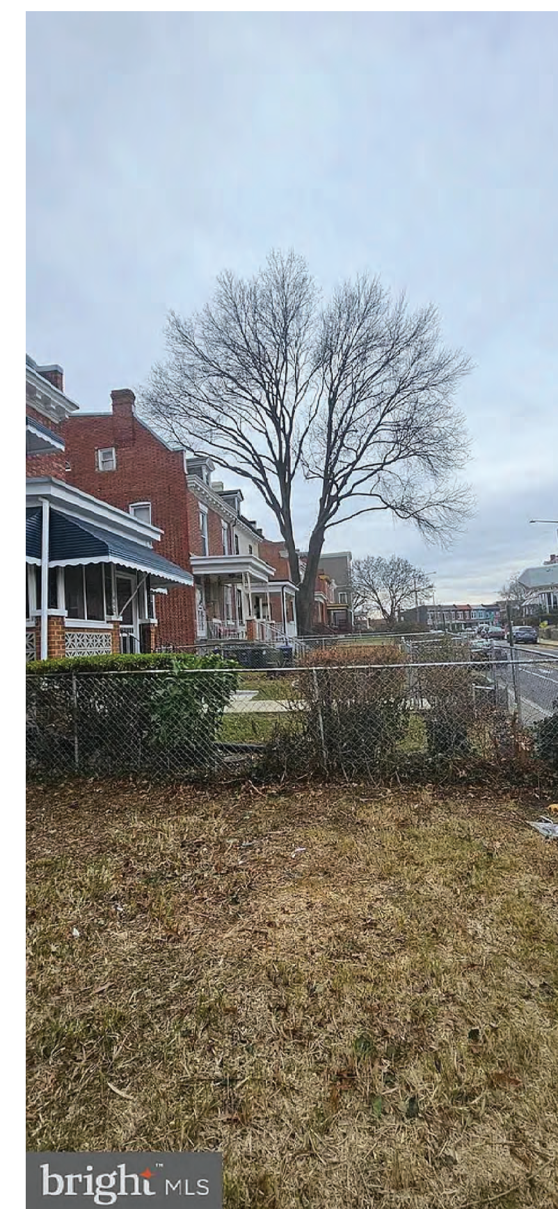
WEST VIEW FROM YARD 438 PARK ROAD NW
