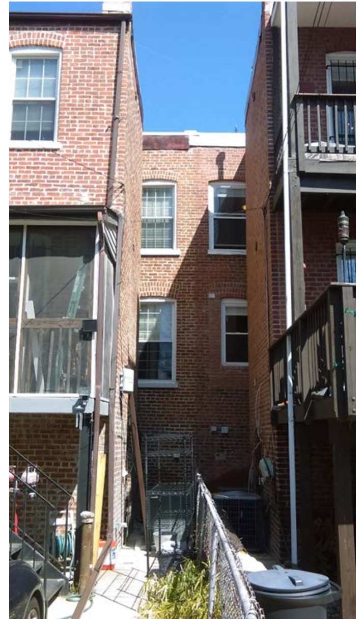
Existing house rear court
