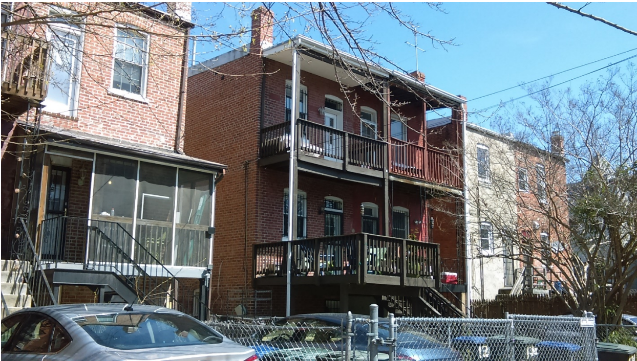
Rear of 122 V ST NW (on left) and houses to its east
