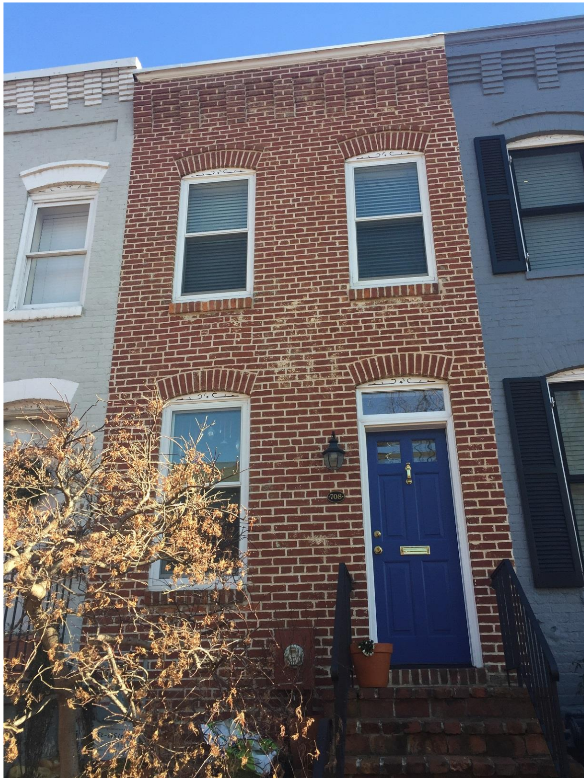
EXISTING FRONT FAÇADE
