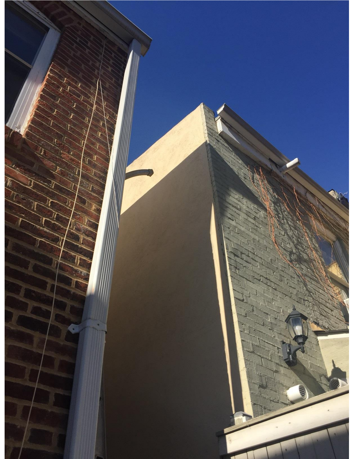
VIEW FROM REAR YARD, LOOKING TOWARD 706 4 TH STREET SE
