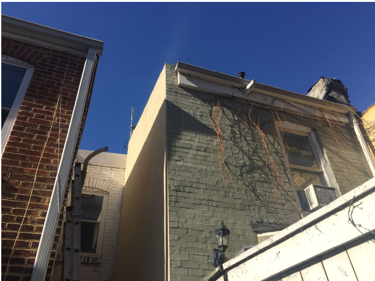
VIEW OF 706 4 TH STREET SE
