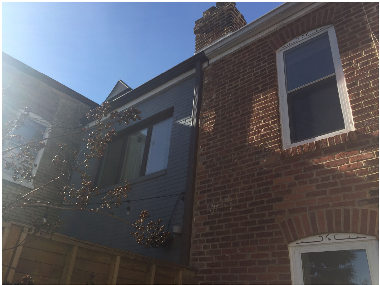
VIEW OF 710 4 TH STREET SE
