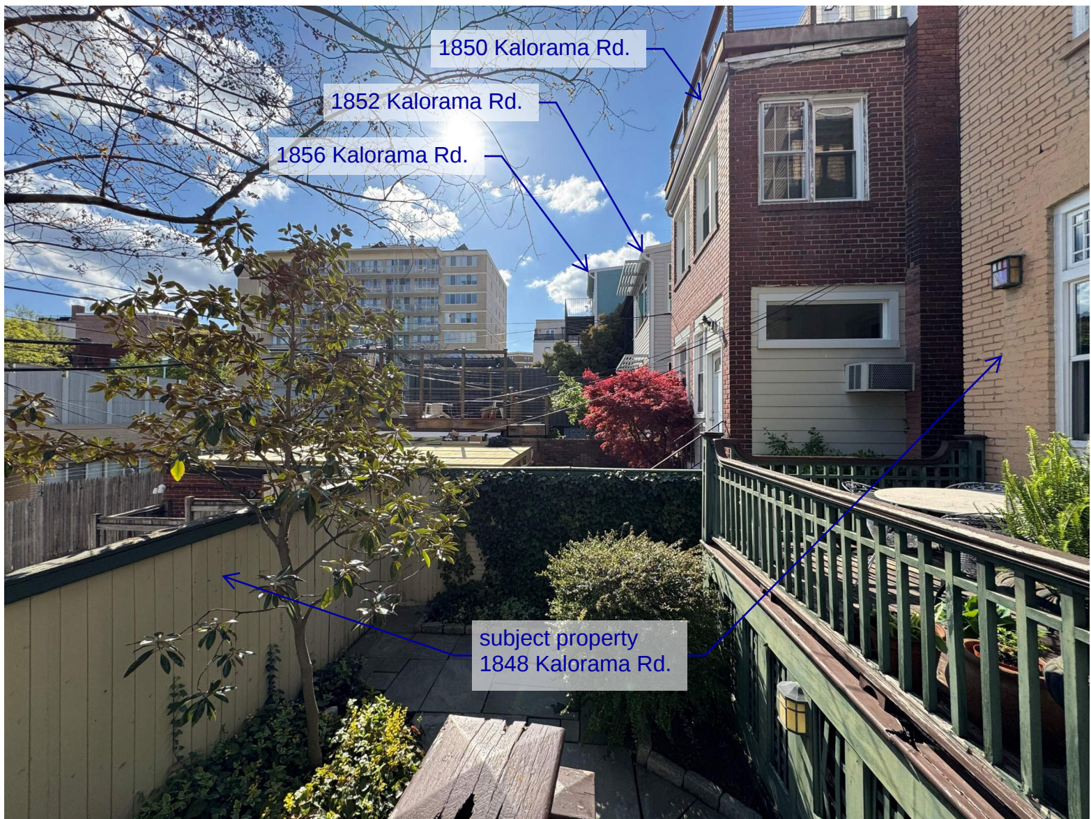
1848 Kalorama Road, NW - Existing Rear Yard Looking West
