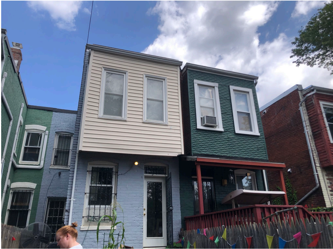
VIEW FROM REAR YARD, LOOKING EAST
