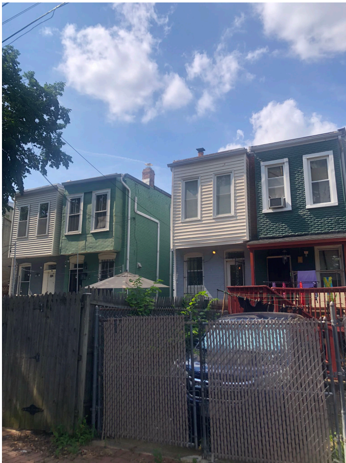
ALLEY VIEW, LOOKING WEST
