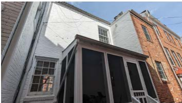
IMAGE #3&4 FROM PATIO - SHOWING THE LOCATION OF THE ADDITION ON THE REAR OF THE HOUSE. LOOKING TOWARDS 2726 O ST NW.
