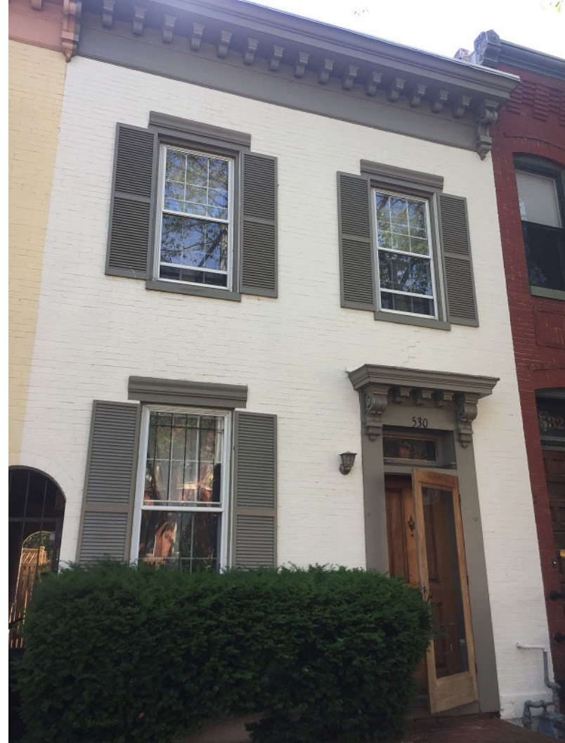
FRONT FAÇADE, 530 11 TH STREET SE
