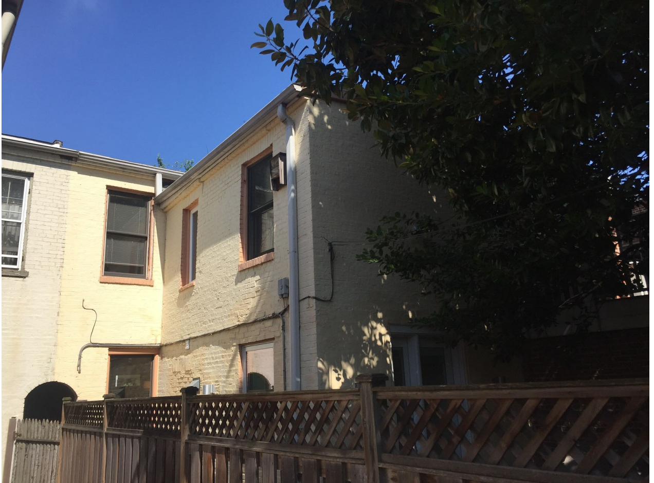
VIEW TOWARDS 528 11 TH STREET SE
