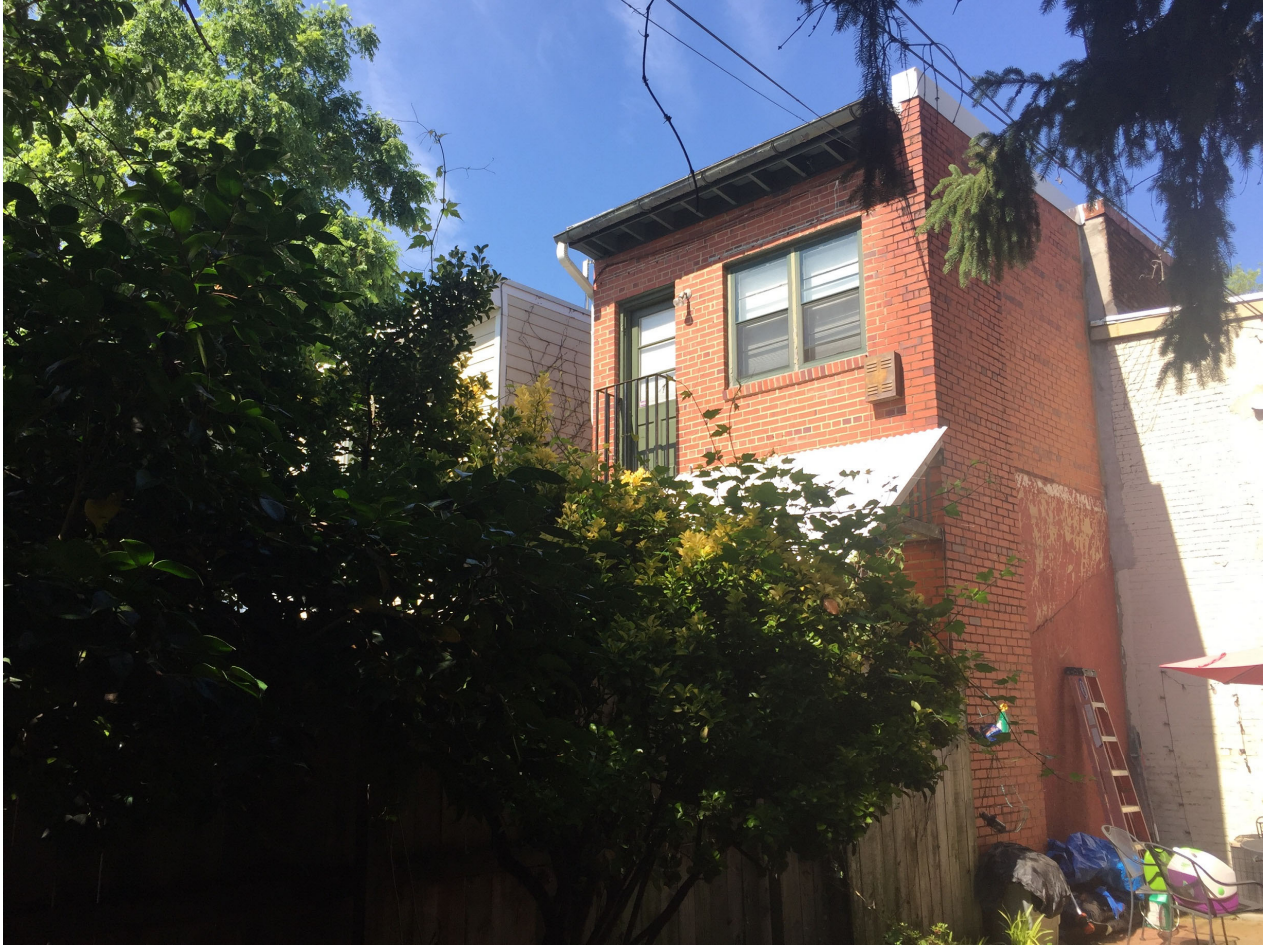
VIEW TOWARDS 532 11 TH STREET SE
