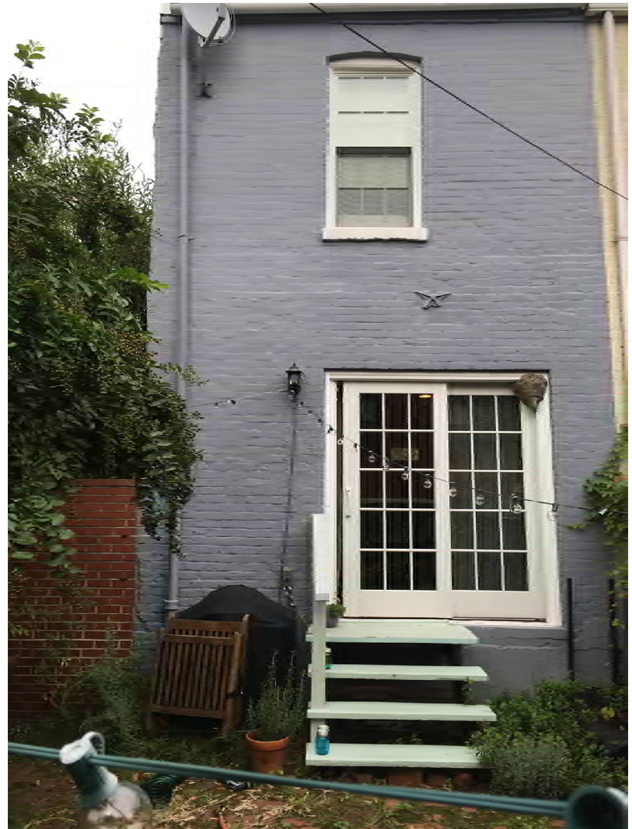
EXISTING REAR FACADE
