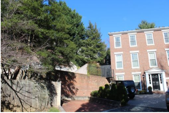
VIEW C: LOOKING NW FROM SOUTH NEIGHBOR
