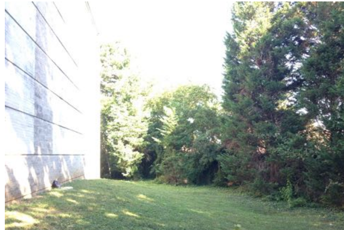
VIEW A: SOUTH ELEVATION LOOKING EAST
