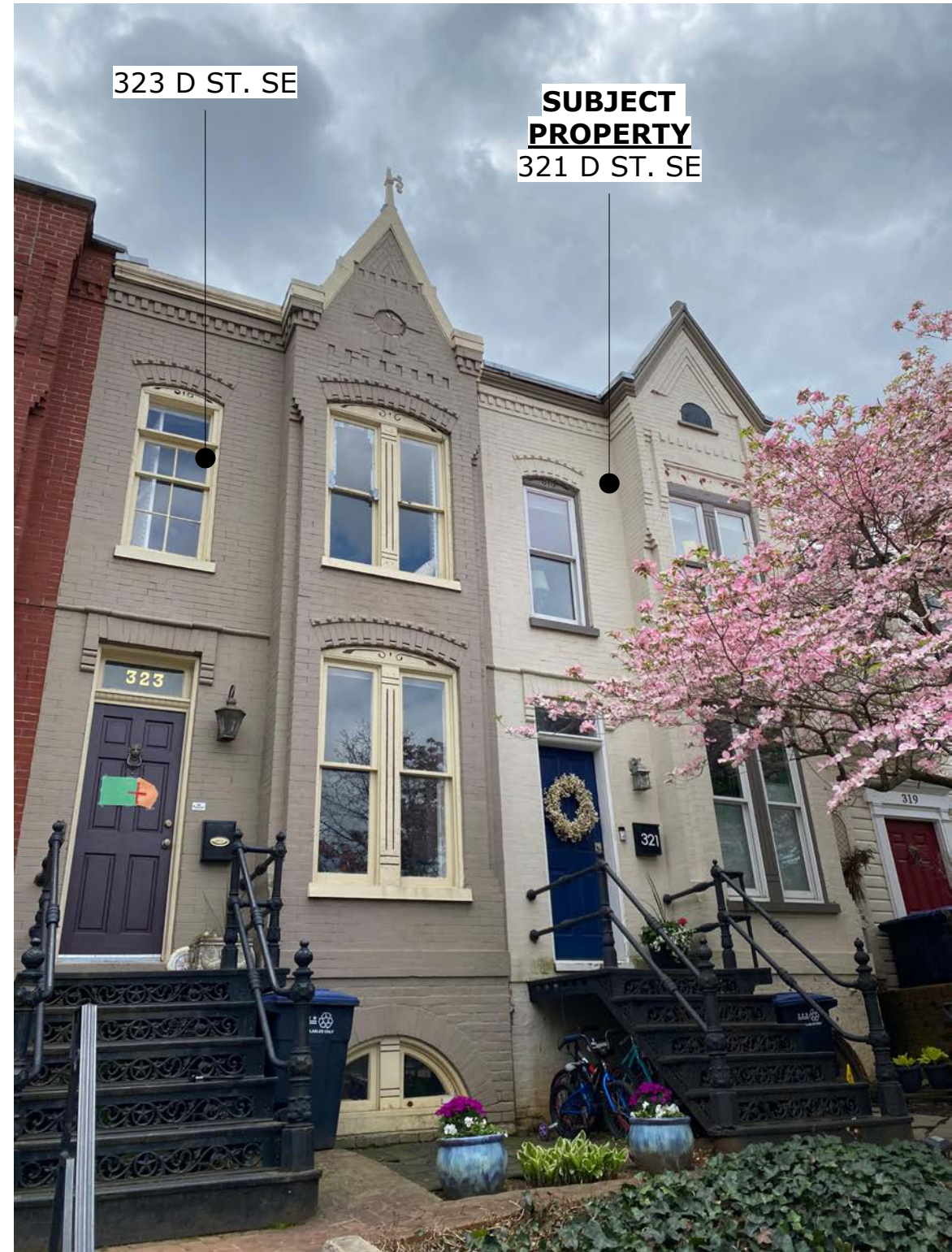
EXISTING FRONT FACADE
