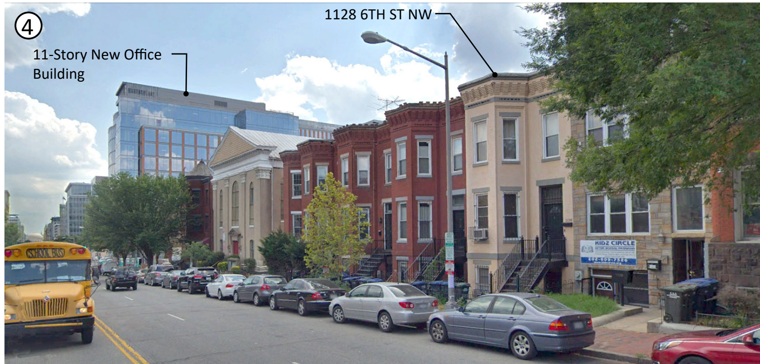
South-West View of 6th Street
