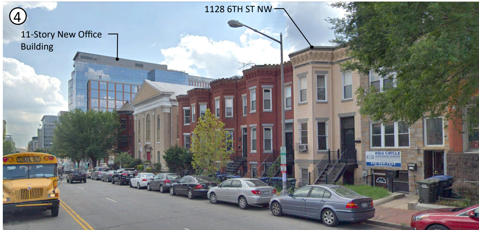
South-West View of 6th Street
