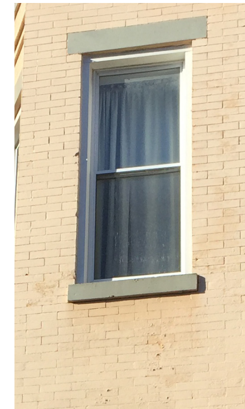
EXISTING PAINTED BRICK- EXISTING PRECAST WINDOW- SILL AND LINTEL
