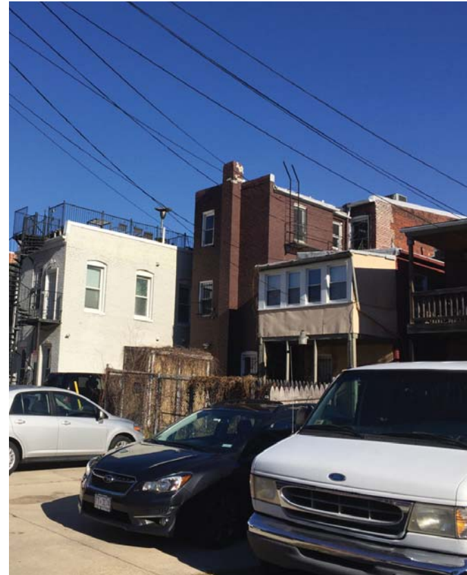
Rear Facade and Alley
