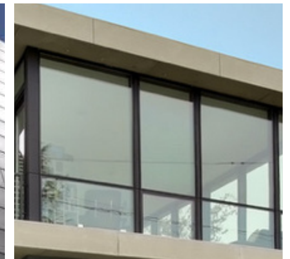
VERTICALLY COMPOSED METAL CLAD WINDOWS- ON ADDITION
