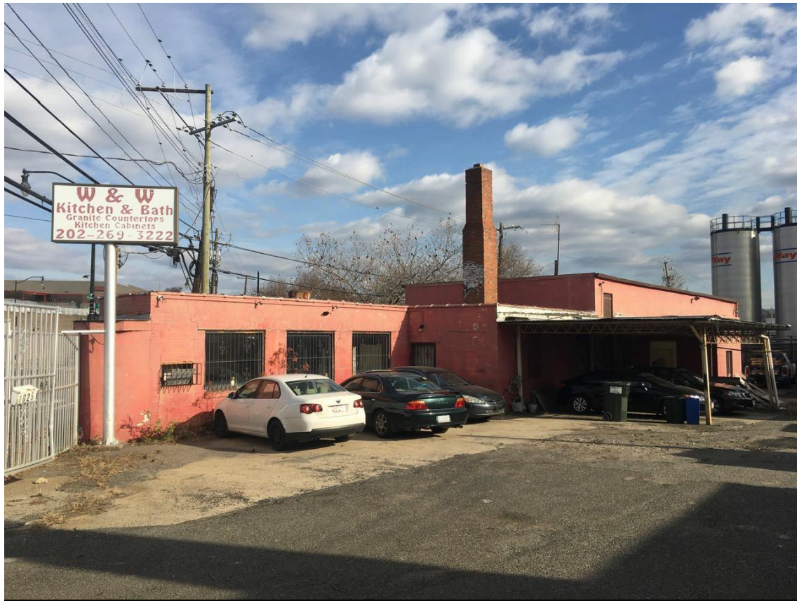
VIEW SOUTH FACADE
