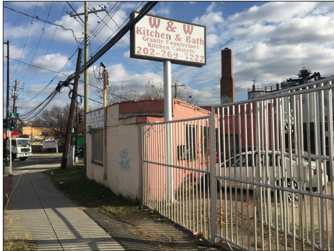
VIEW WEST FACADE
