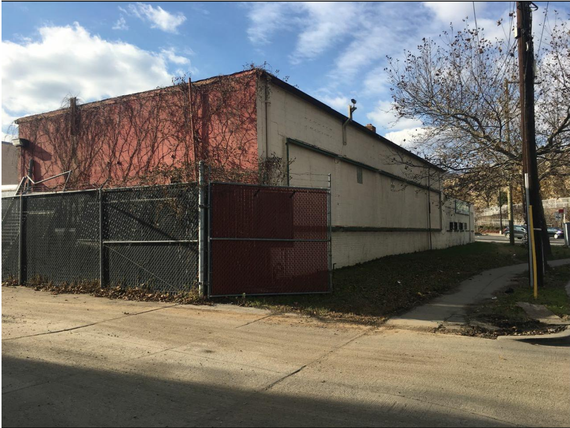
VIEW EAST FACADE
