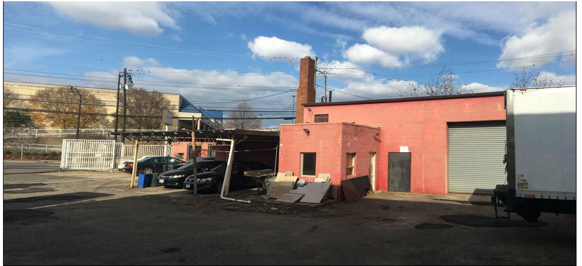
VIEW SOUTH FACADE
