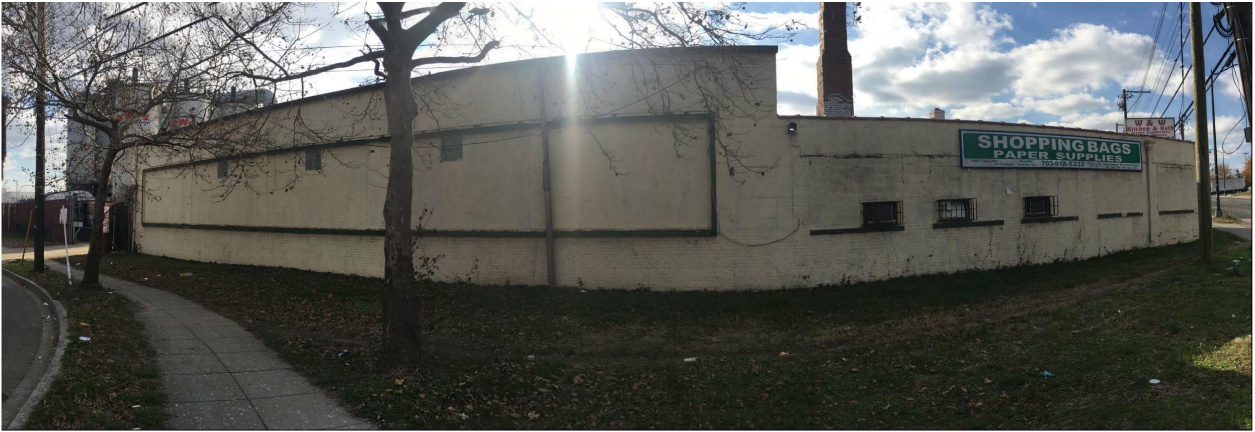
VIEW NORTH FACADE
