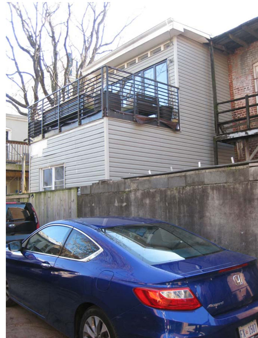
REAR OF 1003 P ST. NW
