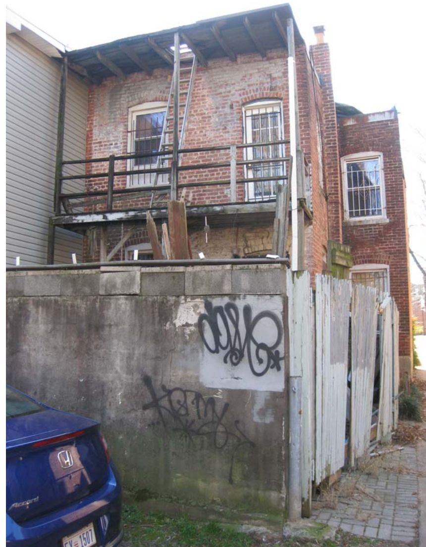
REAR OF 1005 P ST. NW
