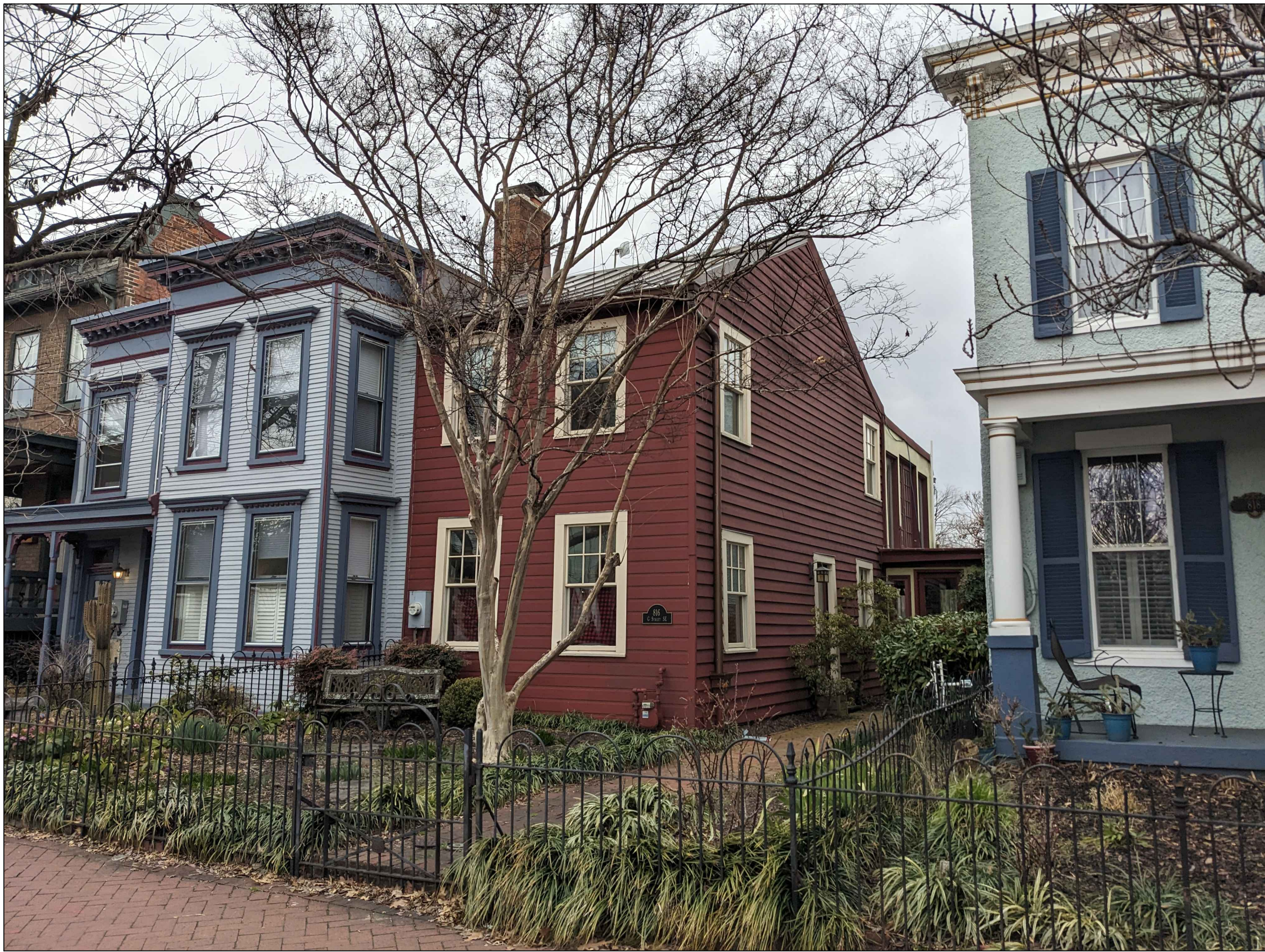
EXISTING FRONT FACADE, FROM SIDEWALK
