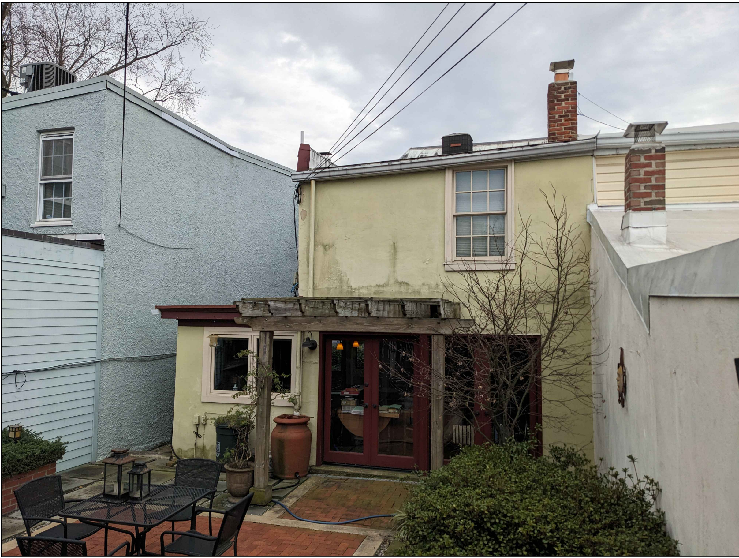
EXISTING REAR FACADE, FROM REAR YARD
