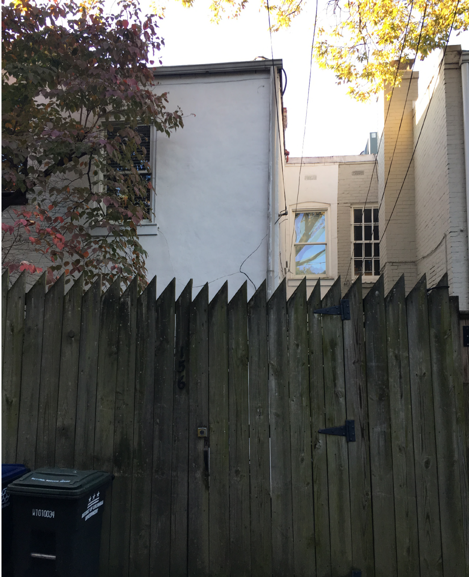
Rear View (from Alley) of 156 Duddington Place SE
