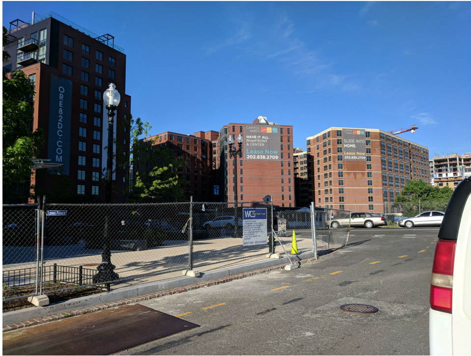
VIEW FROM EXISTING H STREET
