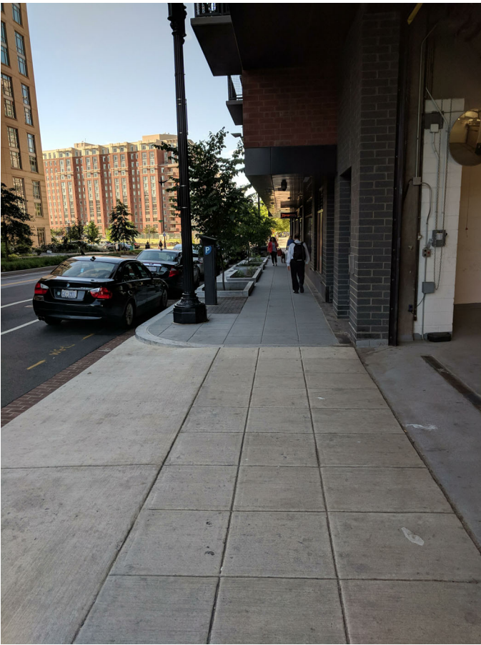
ORE 82 SIDEWALK (LOOKING SOUTH)
