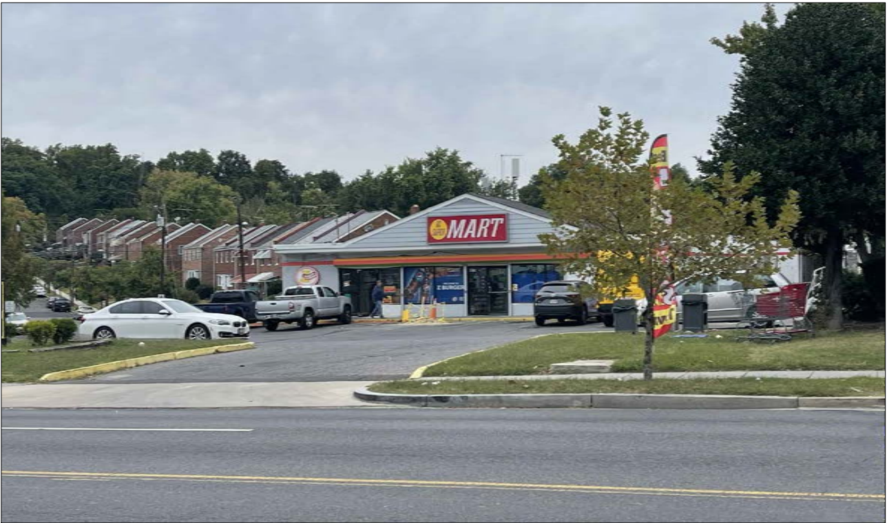
EXISTING SITE IMAGE
