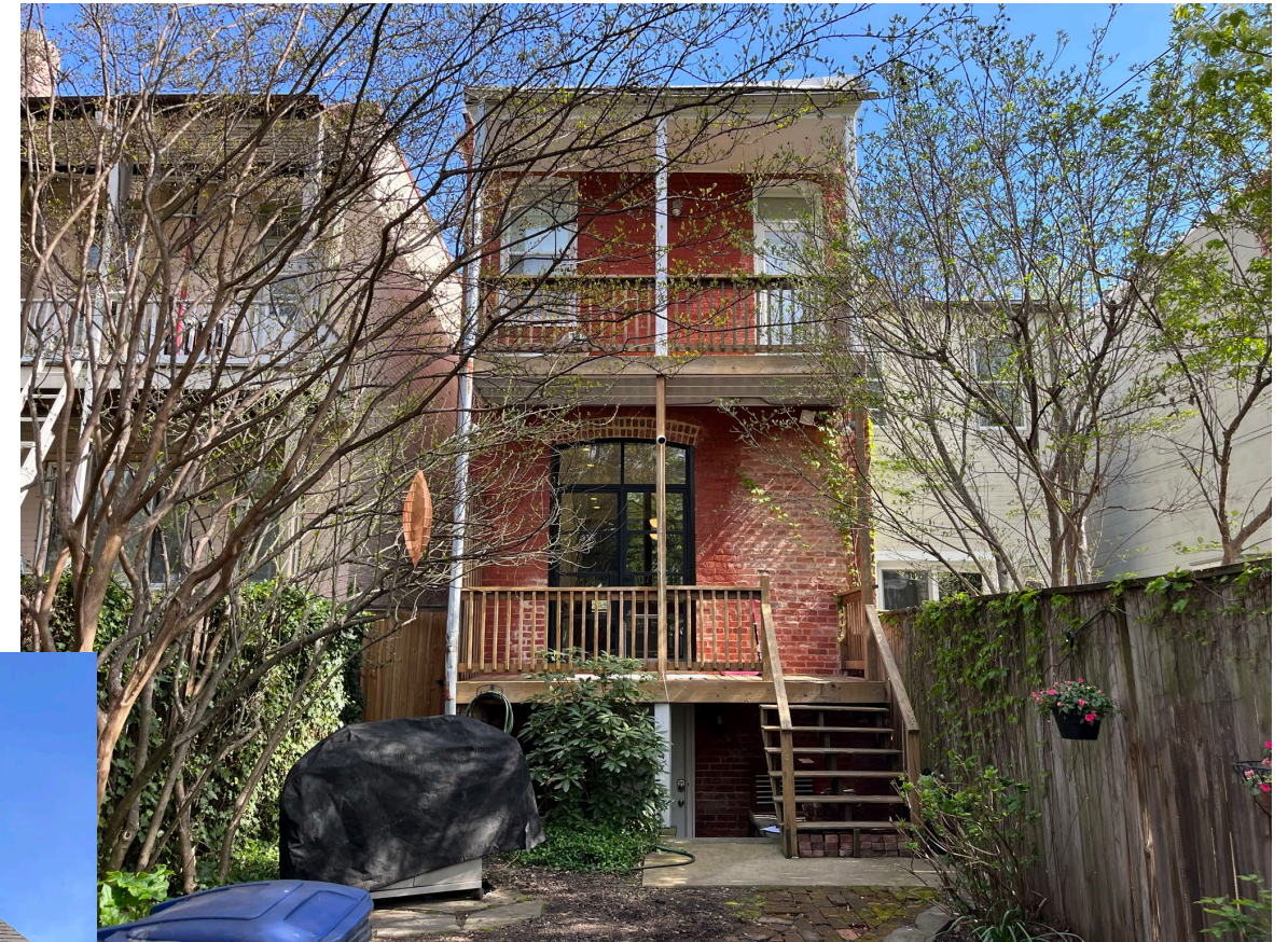
View from rear yard towards 718 N. Carolina Ave SE
