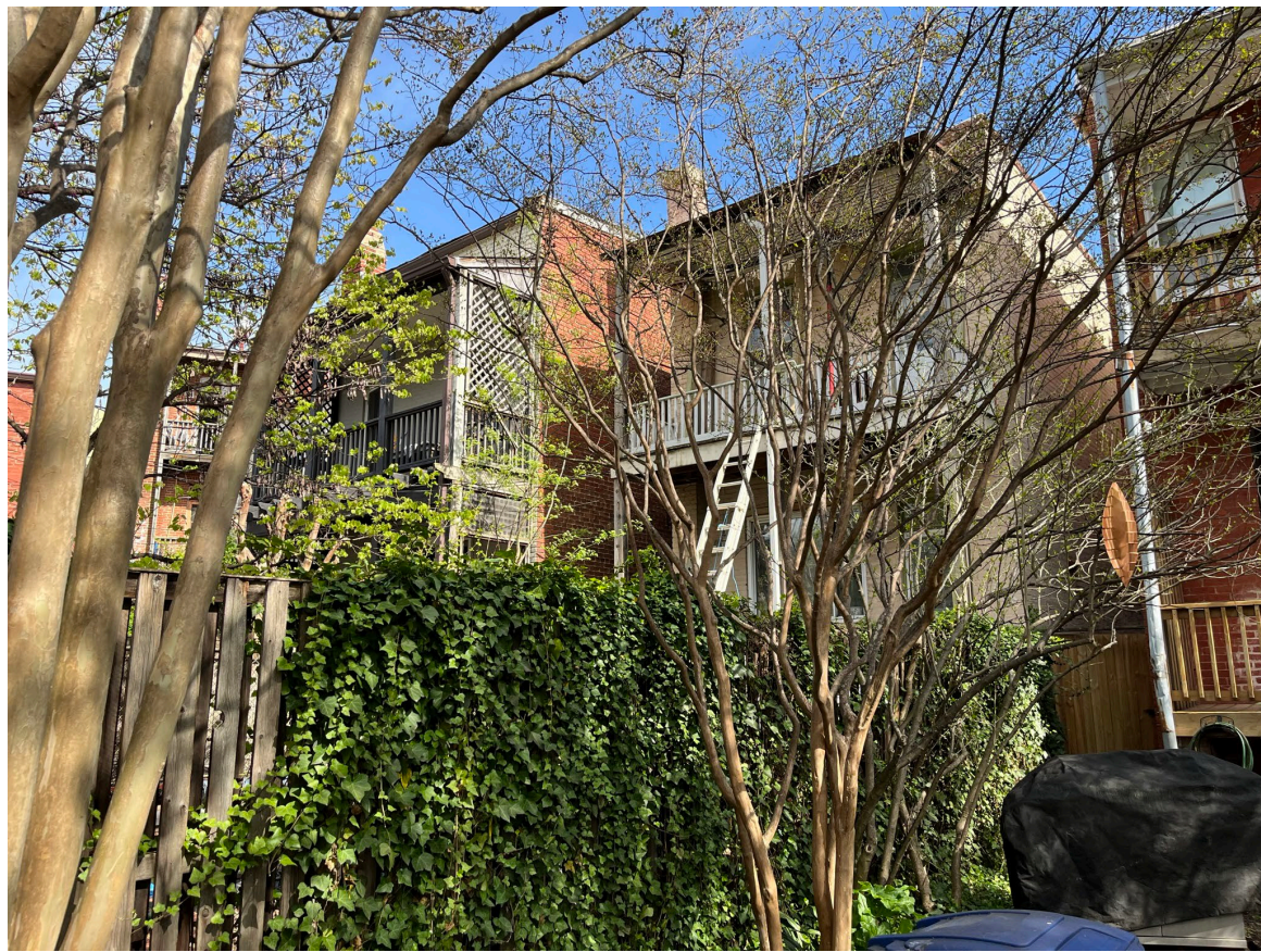
View from rear yard towards 720 N. Carolina Ave SE
