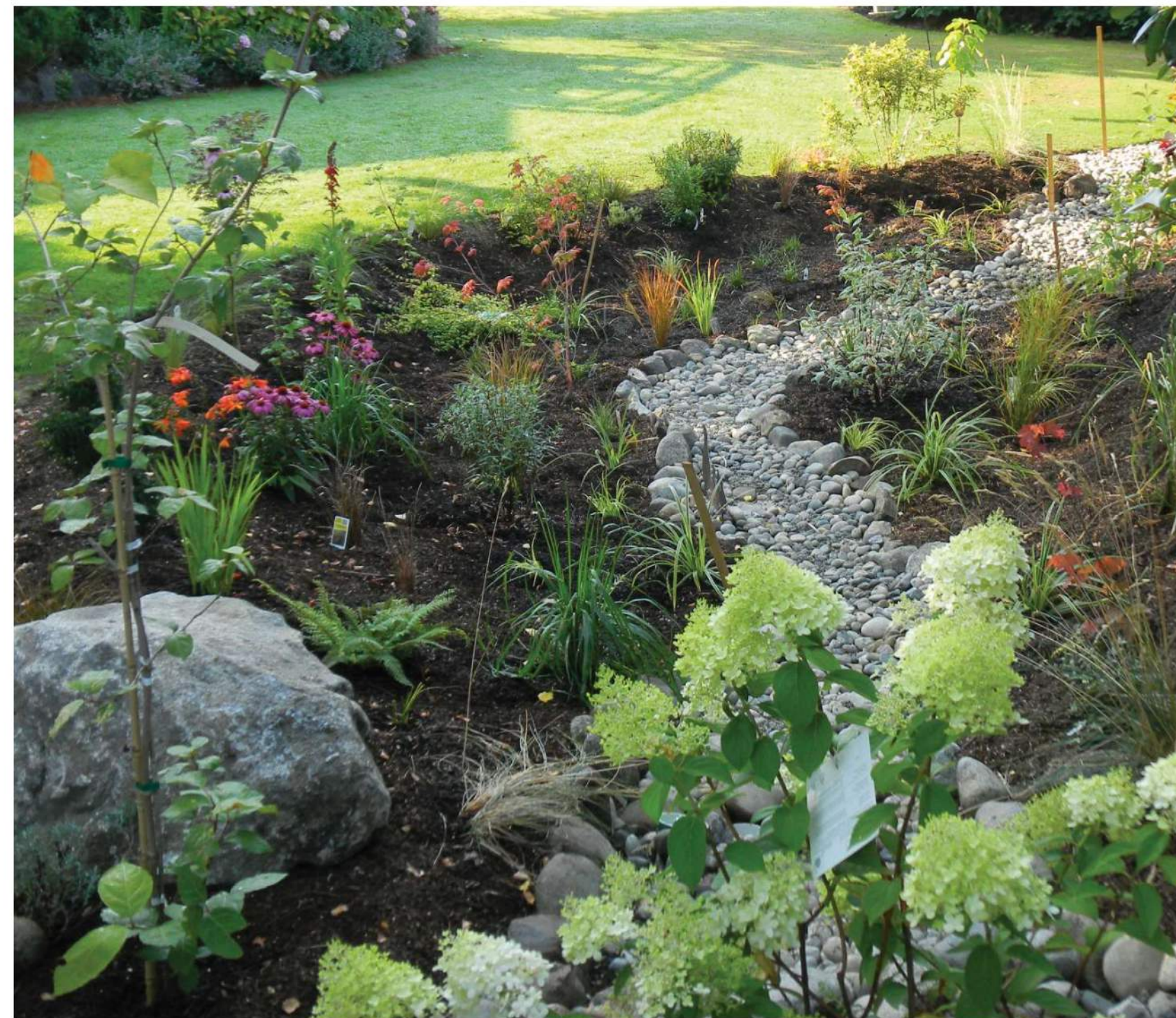
bioretention / stormwater management
