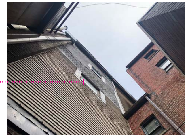
VIEW OF ADJACENT WINDOWS TO NORTH
