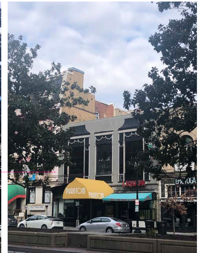
BUILDING TO WEST
