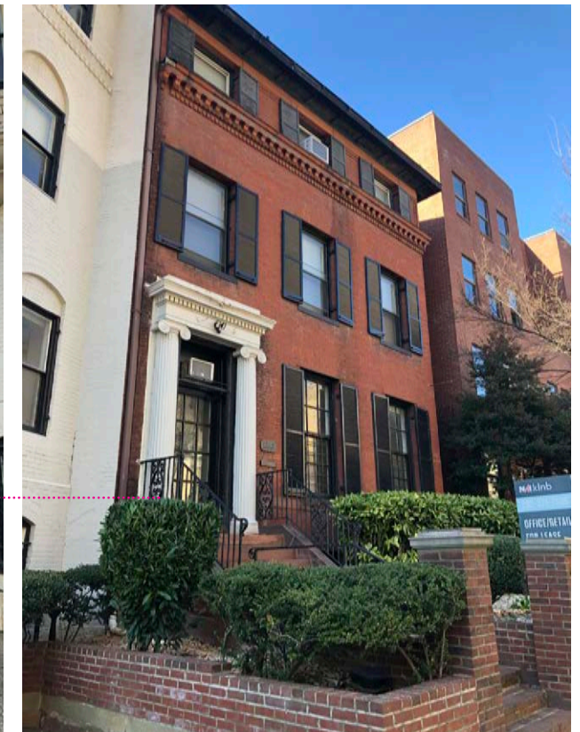
BUILDING TO NORTH
