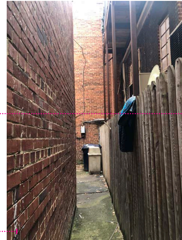
FROM BEHIND 2 STORY STAIR ENCLOSURE LOOKING SOUTH TO REAR COURTYARD
