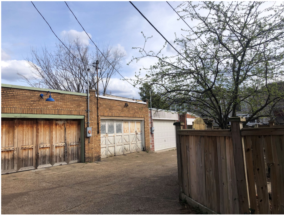
VIEW FROM EXISTING ALLEY, LOOKING SOUTH
