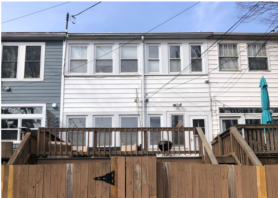
REAR FAÇADE VIEW FROM ALLEY
