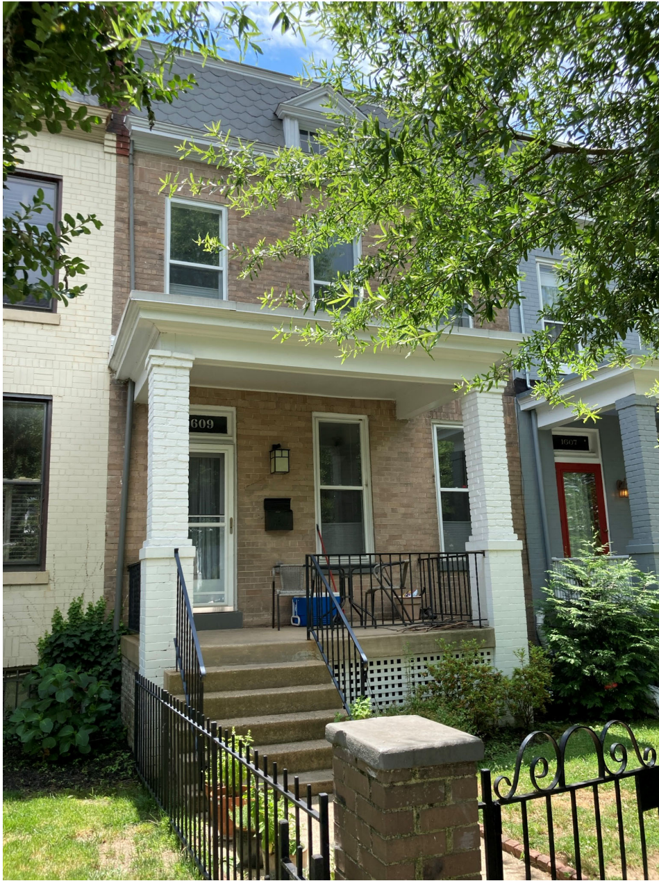
EXISTING FRONT FACADE
