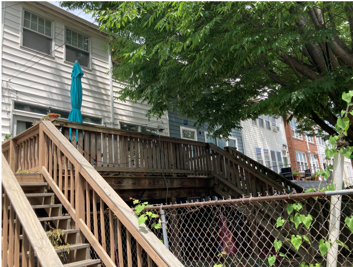
REAR FAÇADE, LOOKING EAST
